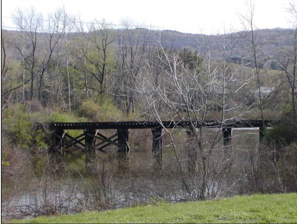
**Figure 9. Franklin Creek - Alternative 2 - Typical Timber Railroad Bridge**
