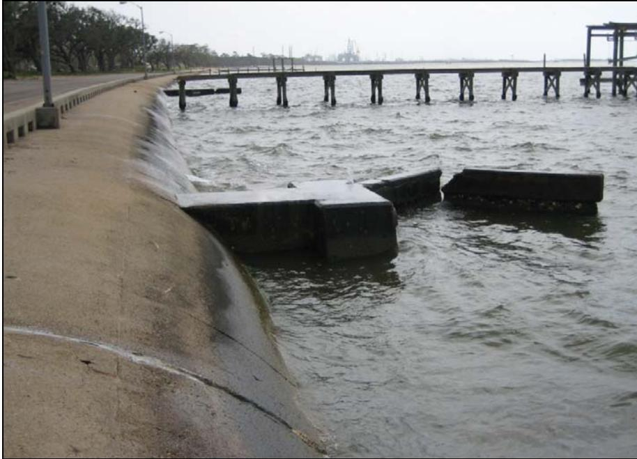
**Figure 5. Concave Seawall, Culvert Outfall, and Pier, Looking East. Beach Boulevard is to the Left.**
