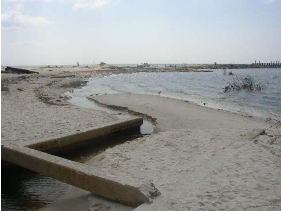
**Figure 5. Looking towards location of destroyed marsh. Approximately 100 feet of erosion in the vicinity of the marsh occurred during Katrina. 3 April 2006 photo**
