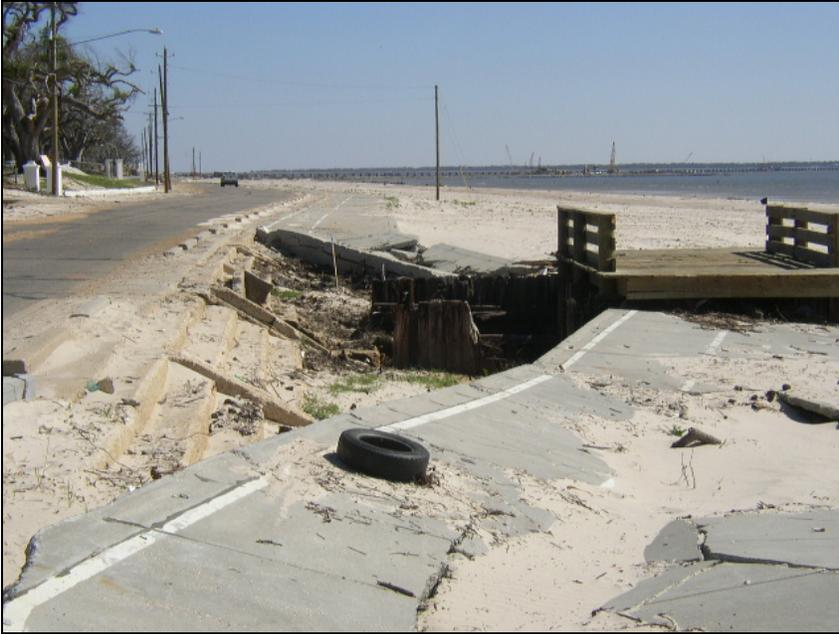
**Figure 4. Damaged pathway, drainage channel outlet, and outlet bridge, near Waveland.**
