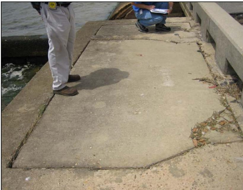
**Figure 10. Intact Cap on West End of Cellular Concrete Box Seawall.**
