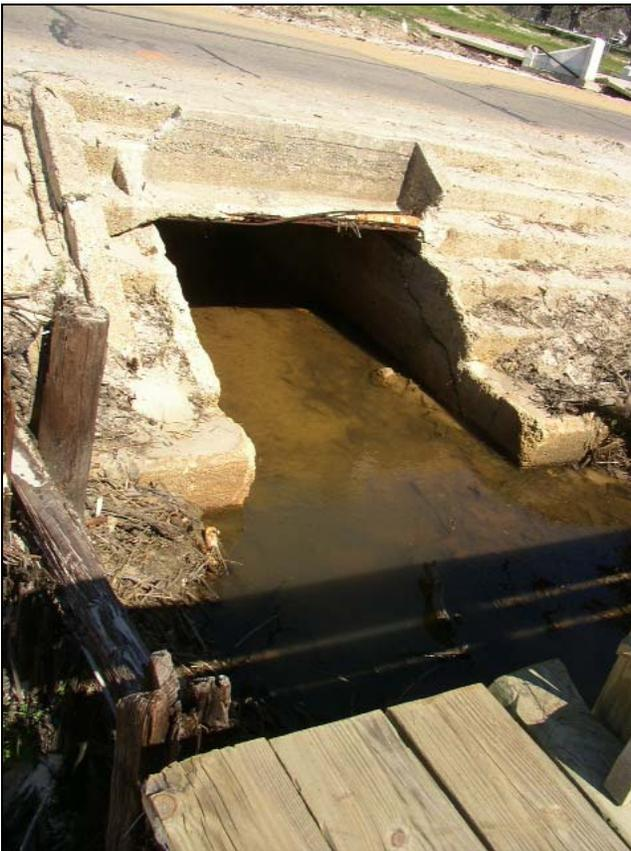
**Figure 5. Close-up of outlet featured in Figure 5. Channel is choked with sand, channel confinement structure destroyed.**
