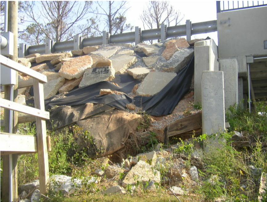
**Figure 6. Timber Wall Failure at North Abutment**
