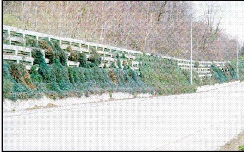
**Figure 9a. Example Landward Barrier, Railroad Barrier Concept**
