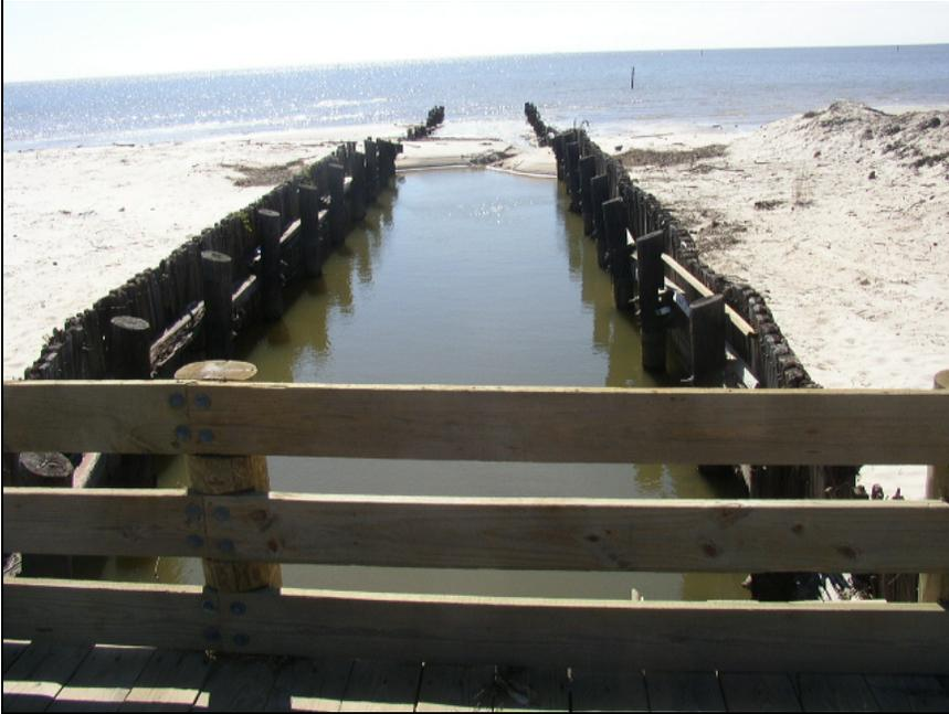
**Figure 6. Channel outlet. Outlet is breached, extension walls are damaged, and outlet is choked with sand.**
