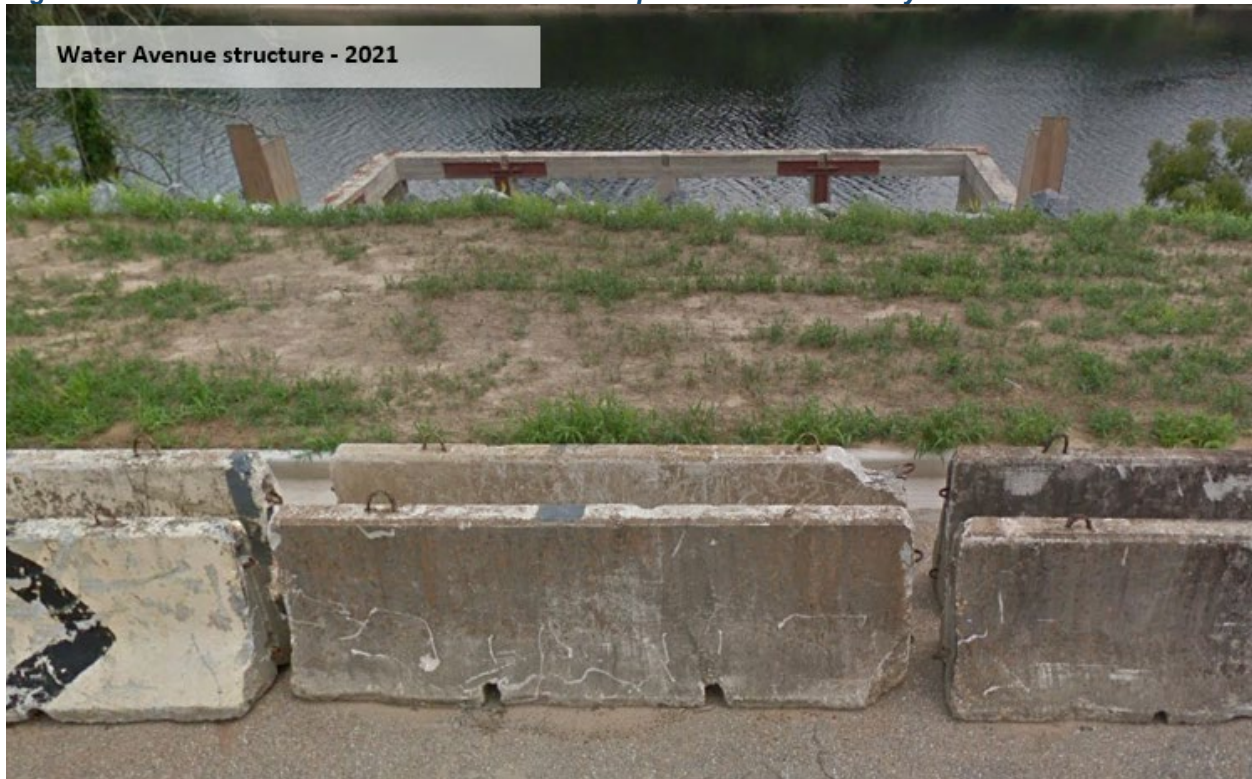
Figure C-11: Structure on Water Avenue that collapsed due to instability
