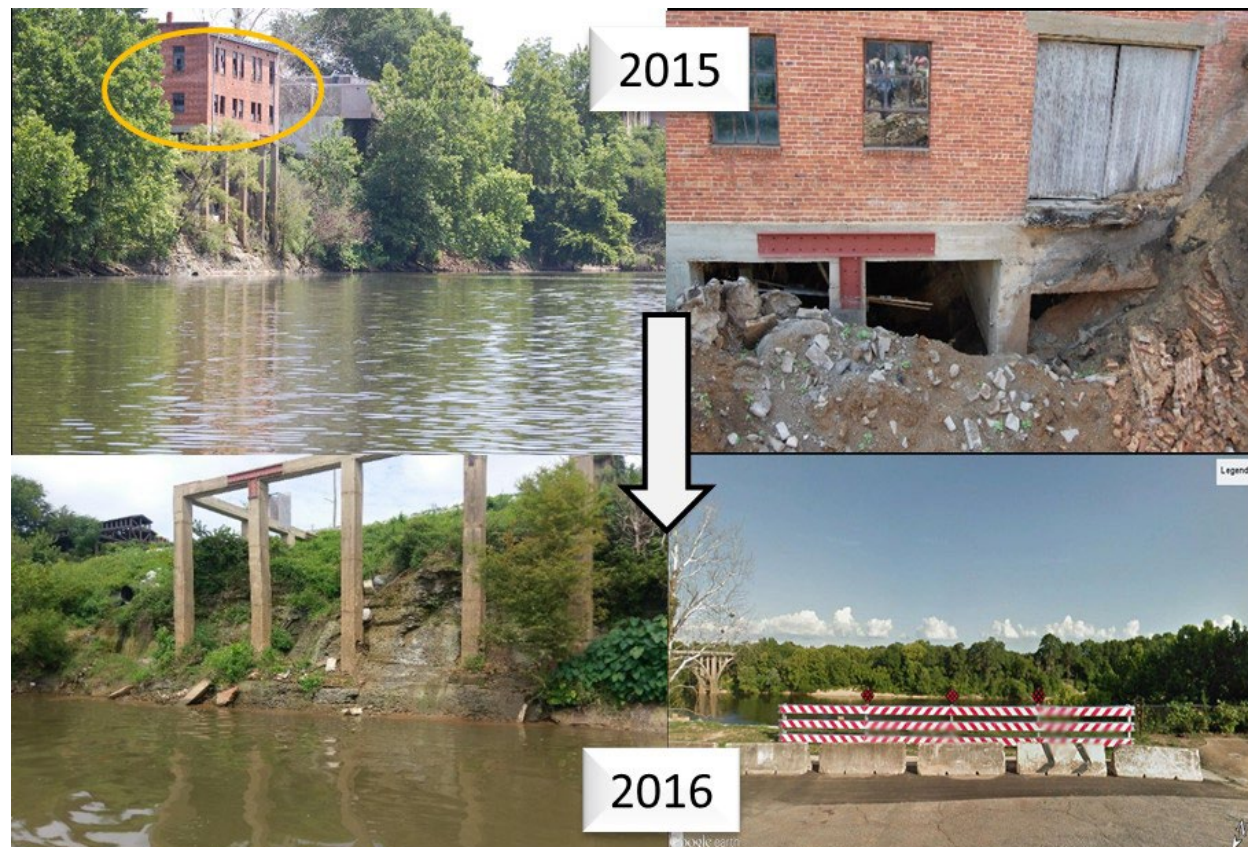
Figure 3: Structural Demolition Due to Bank Erosion in 2016
