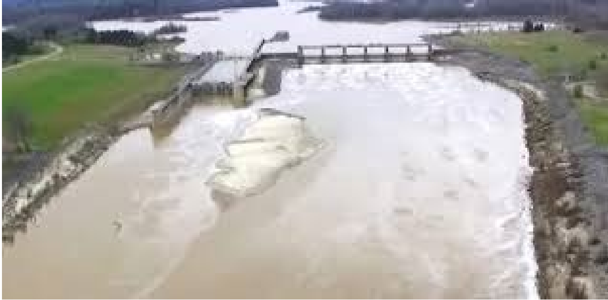
Figures 2 & 3. Severe rain events can result in significant shoaling on the Tombigbee Waterway
