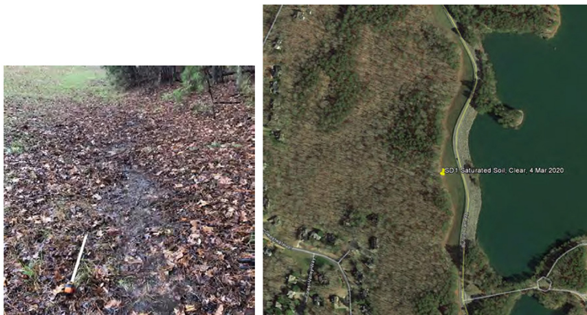
Figure 1 Figure 7: View S along the toe of Saddle Dike 1, saturated soil and leaf debris; clear water was observed at toe (photo taken 3/4/20 at location 34.171133, -84.078565; refer to aerial), for a 100 ft. length along toe, and for a distance 8 ft. perpendicular to toe near central portion of the saturated soil. Tape measure is extended 2.0 ft. Upper pool at EL +1075.24 ft. is left of the left photo. The full 2,300 ft. length of SD1 is shown in the photo on the right (imagery date 3/16/19). SD1 structural height is 36 ft.
