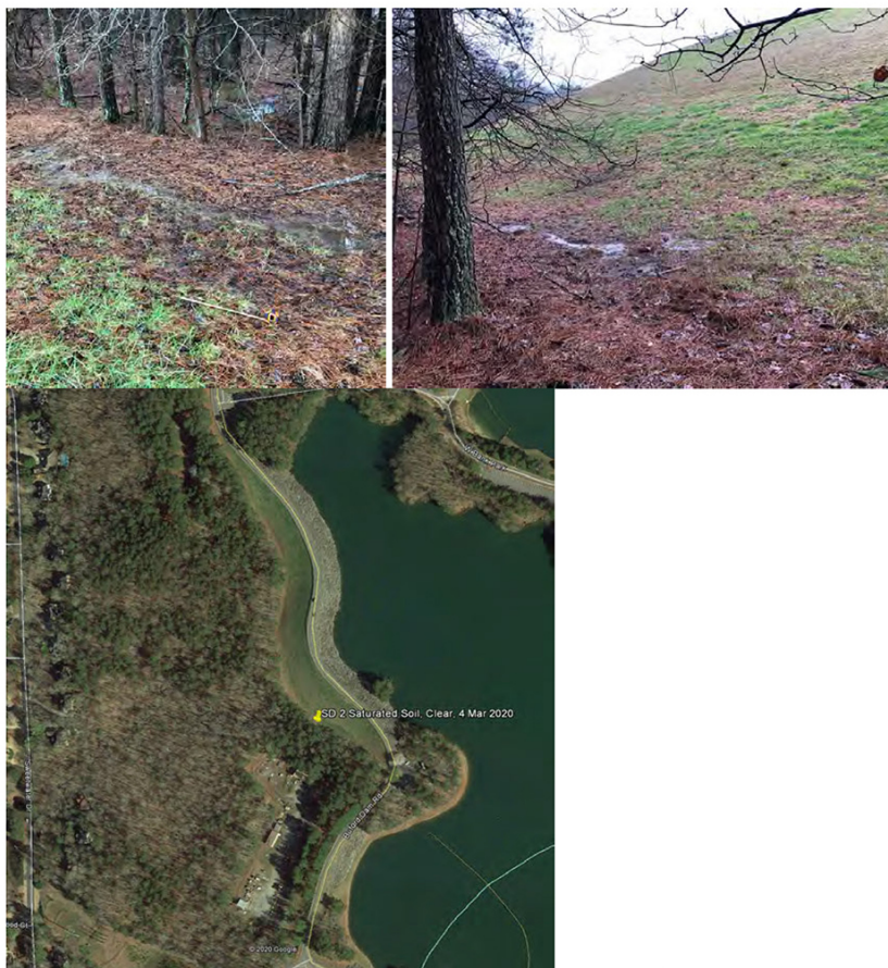
Figure 2 Upper left is view S and below the toe of Saddle Dike 2; upper right is view NW, saturated soil and leaf debris; clear water was observed at toe (photo taken 3/4/20 at location 34.165389, -84.076825; refer to aerial), for a 150 ft. length along toe, and for a distance 10 ft. perpendicular to toe near central portion of the saturated soil. Tape measure is extended 2.0 ft. Upper pool at EL +1075.24 ft. is left of the left photo. The full 2,300 ft. length of SD2 is shown in the photo on the right (imagery date 3/16/19). SD2 structural height is 48 ft.
