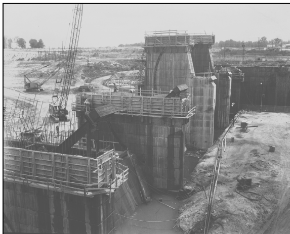
Figure 3-2. Gate Supports, Circa 1961-62
