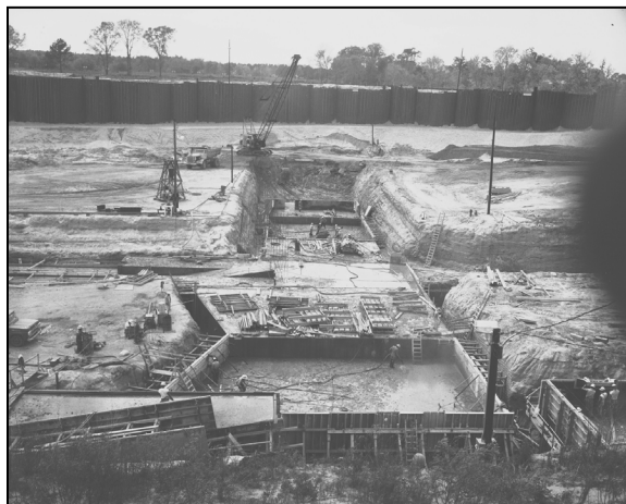
Figure 3-3. Foundation for Miter Gate, Circa 1961-62
