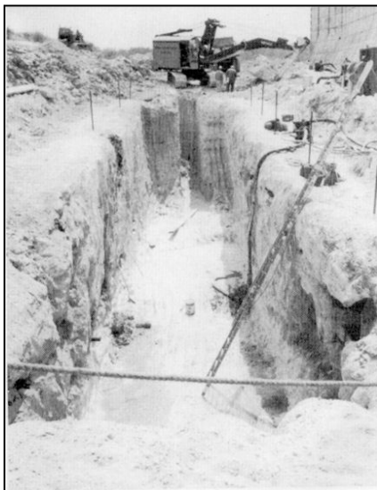
Figure 3-3. Early Excavation to Prevent Seepage
