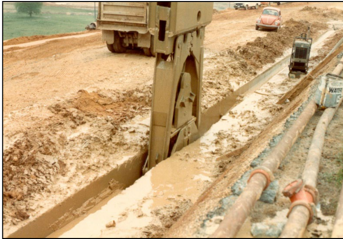
Figure 3-6. Trench Excavation for Cutoff Wall
