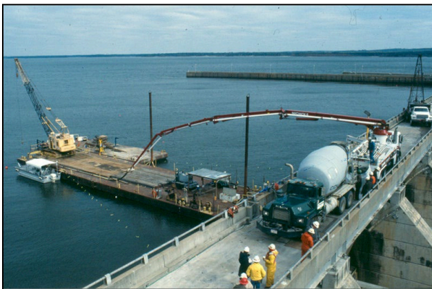
Figure 3-5. Boom Supplying Grouting Operation
