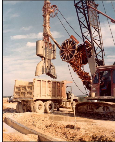
Figure 3-7. Cutoff Wall Construction
