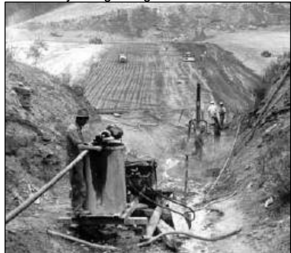
Figure 3-1. Foundation work at Buford Dam (Circa 1950-51)
