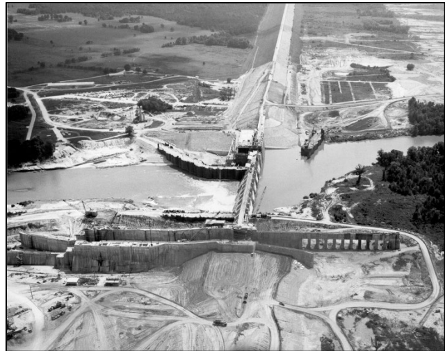
Figure 3-2. Construction at Walter F. George Lock and Dam (Circa 1962)
