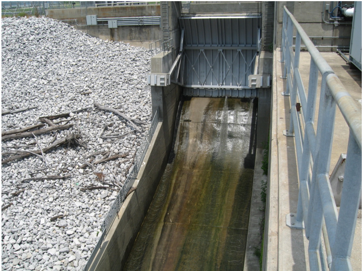
Figure 3-1. Trash Gate at Millers Ferry Project
