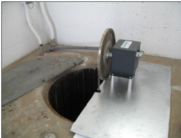
Figure 5-1. Typical Encoder with Wheel Tape for Measuring the River Stage or Lake Elevation in Stilling Well
