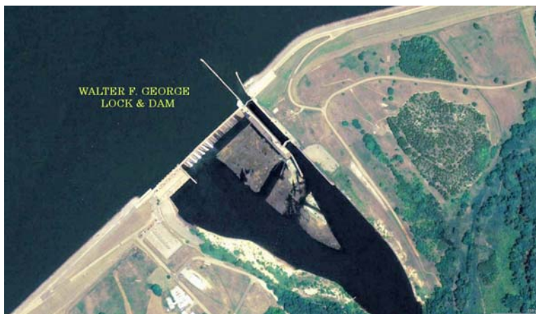
Figure C-30. Walter F. George Dam
