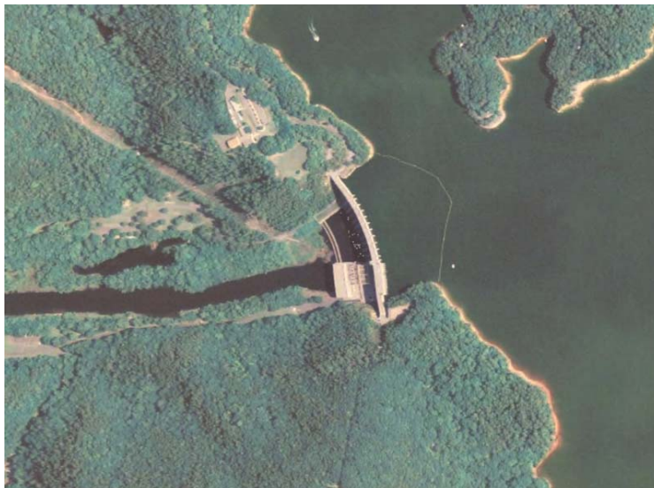
Figure B-5. Allatoona Dam
