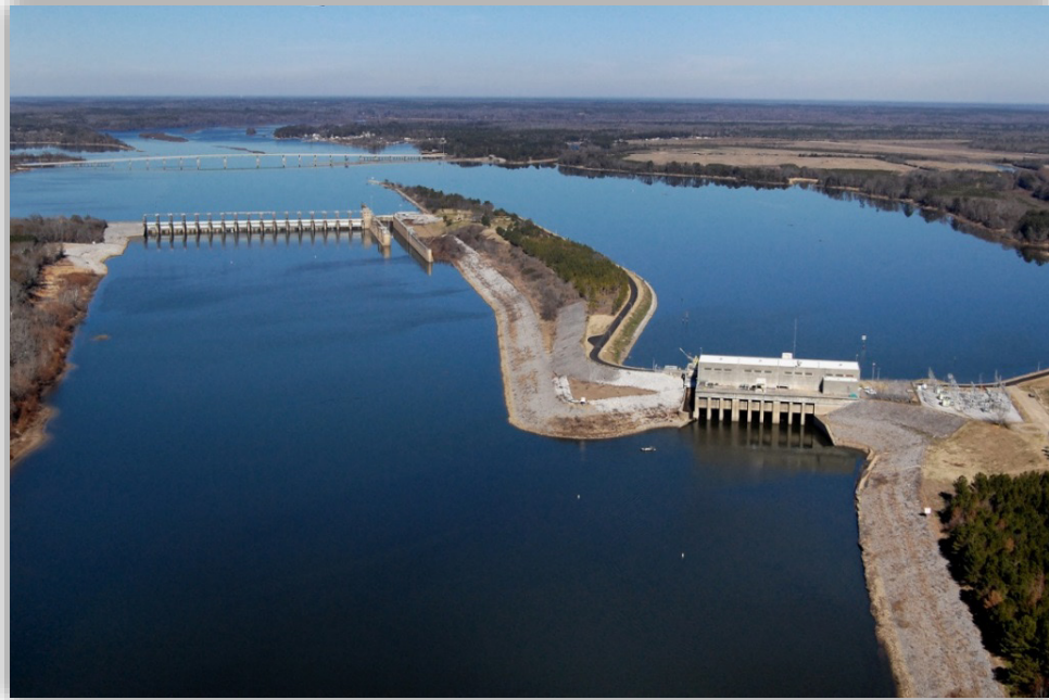
Figure 2-5 Millers Ferry Lock and Dam
