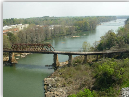
Figure 4-15 Tallapoosa River at Tallassee, Alabama
