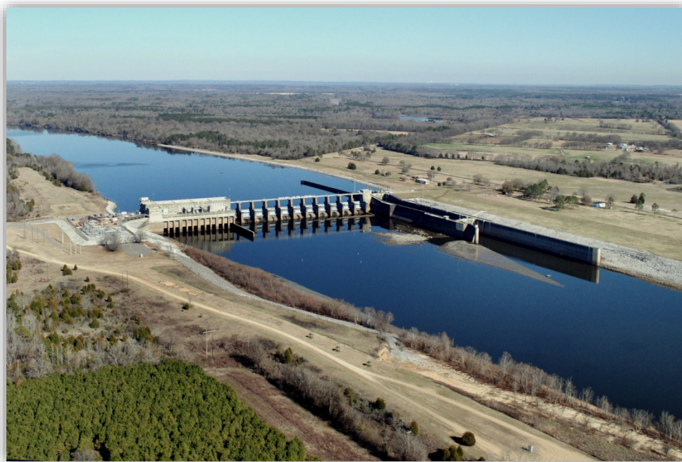
Figure 2-4 Robert F. Henry Lock and Dam
