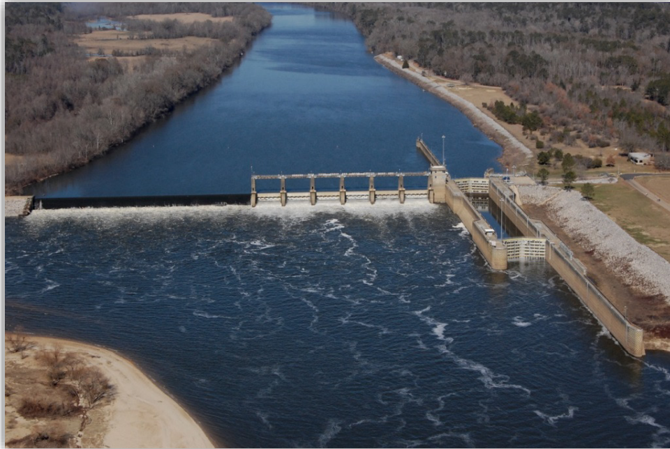
Figure 2-6 Claiborne Lock and Dam
