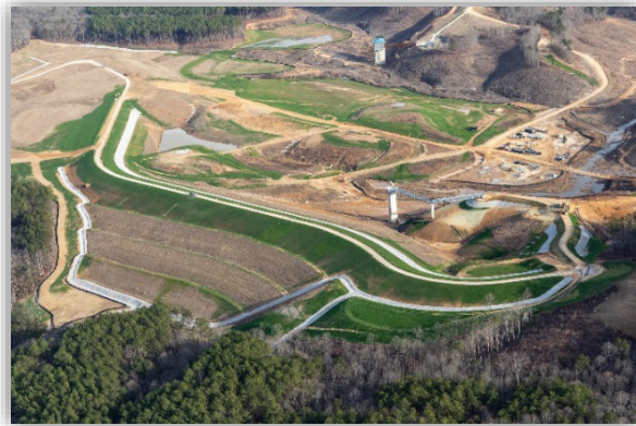
Figure 2-20 Richland Creek Dam
