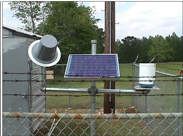
Figure 5-2 Typical Field Installation of Precipitation Gage
