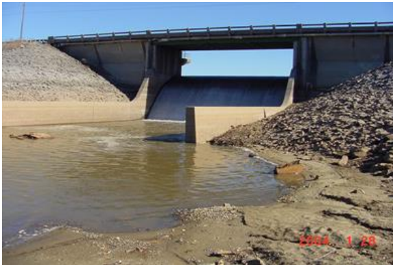
Figure 2-7 Acworth Sub-Impoundment, Ungated Spillway
