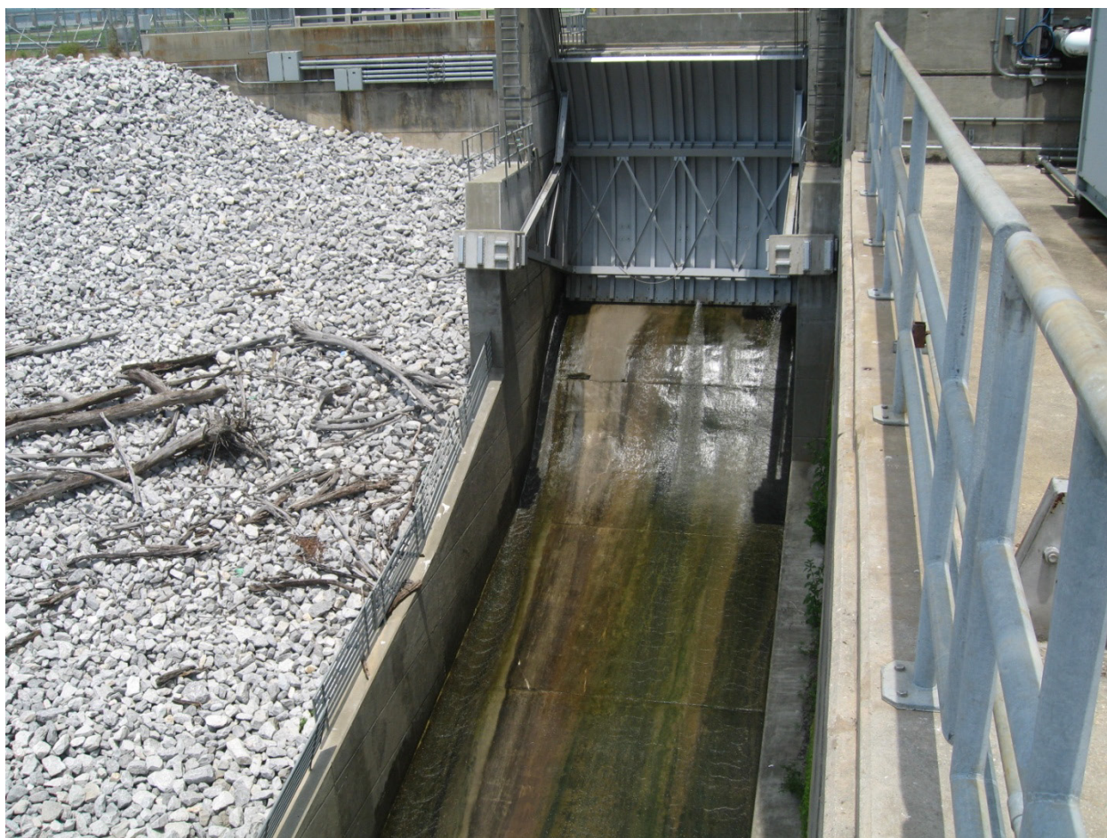
Figure 3-1 Trash Gate at Millers Ferry Project
