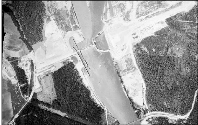
Figure 3-1. Cofferd Dam Protecting the Powerhouse Construction, Circa 1952-53
