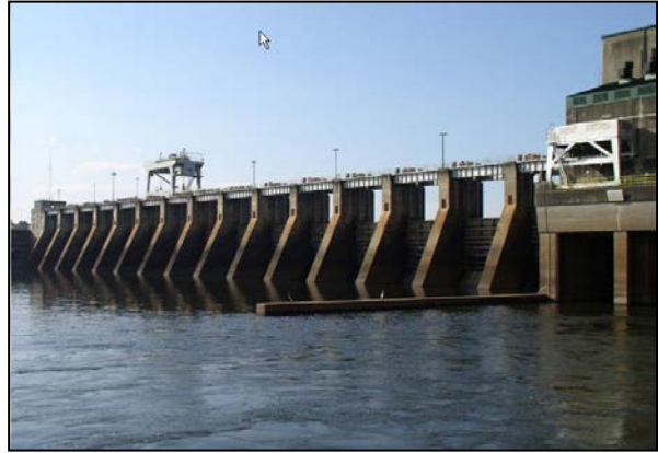
Figure 2-2. Jim Woodruff Spillway Gates
