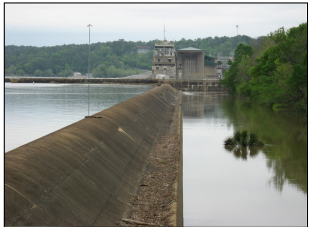
Figure 2-3. Fixed-Crest Spillway without Flow Over the Top
