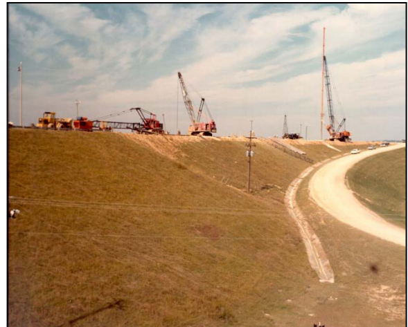
Figure 2-3. Earth dikes during construction of cutoff wall
