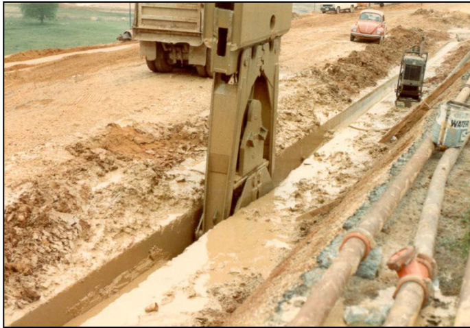
Figure 3-6. Trench Excavation for Cutoff Wall
