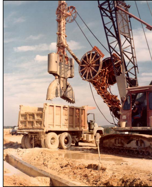
Figure 3-7. Cutoff Wall Construction
