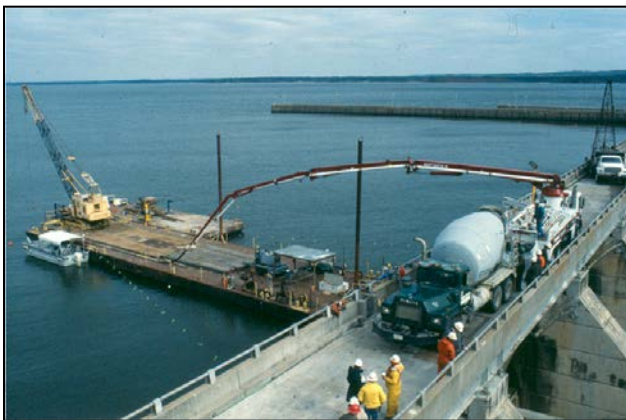
Figure 3-5. Boom Supplying Grouting Operation
