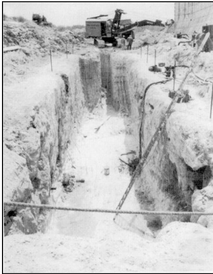
Figure 3-3. Early Excavation to Prevent Seepage
