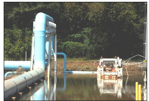
Chattahoochee River flooded the R.M. Clayton Water Reclamation Center. The center is in northwest Atlanta near Cobb County
