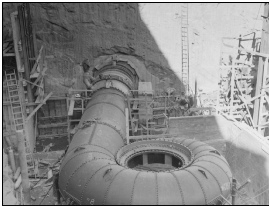
Figure 3-4. Steel Penstock and Scroll Case, 1953
