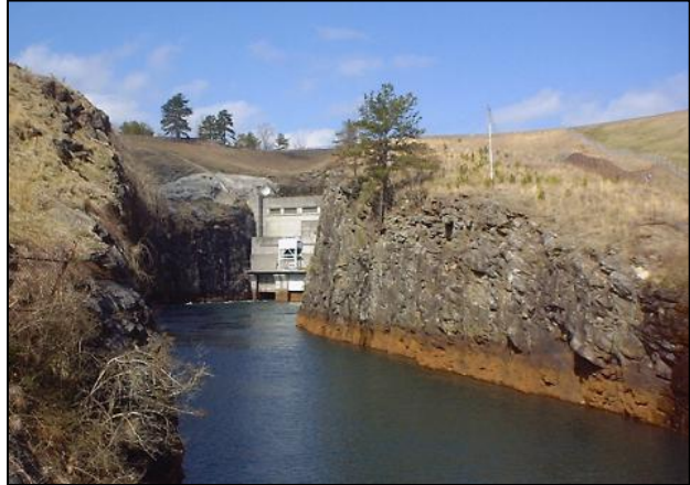
Figure 2-7. Powerhouse and Discharge Channel
