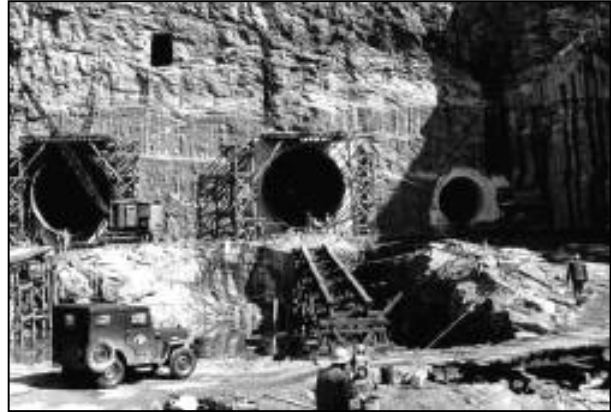
Figure 3-3. Penstock Construction, 1953
