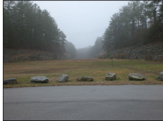
Figure 2-4. Spillway and Uncontrolled Chute
