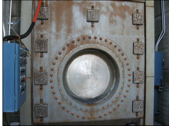
17 Figure 2-6. Broome-type Sluice Gate
