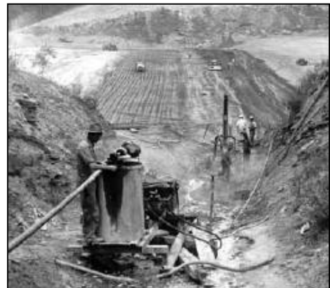
Figure 3-6. Main Dam Construction, 1952
