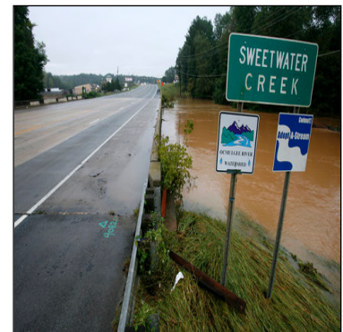
Sweetwater Creek flooding
