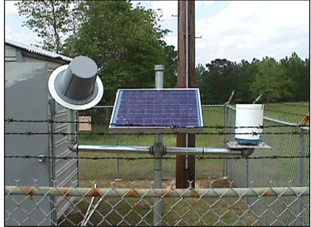
Figure 5-2. Typical Field Installation of a Precipitation Gage
