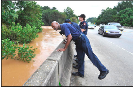
View on MLK Drive. Water was less than 2 feet below the bridge
