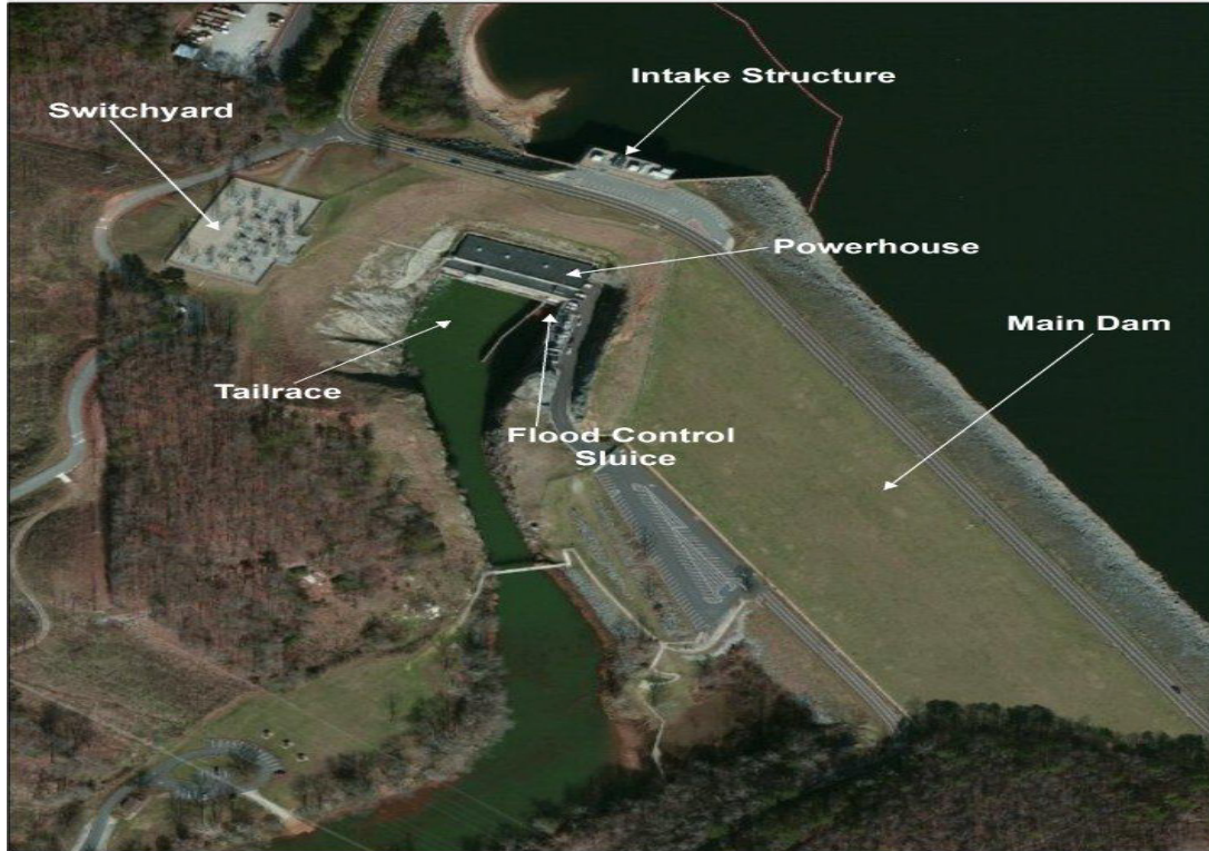
1 2 Figure 2-9. Aerial View of Buford Dam with Physical Components
