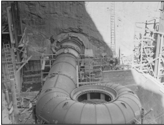
Figure 3-4. Steel Penstock and Scroll Case, 1953
