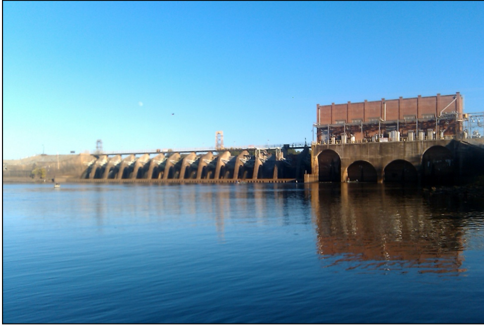
Figure 4-18. Crisp County Dam
