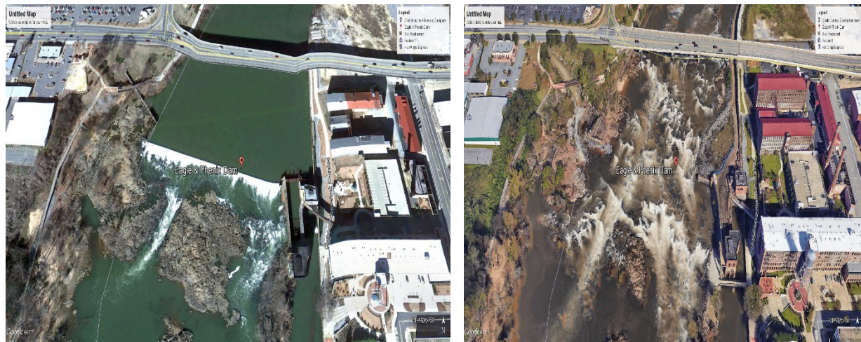
Figure 4-17. Eagle and Phenix Dam Before and After Dam Removal (Photograph courtesy of Google Earth)
