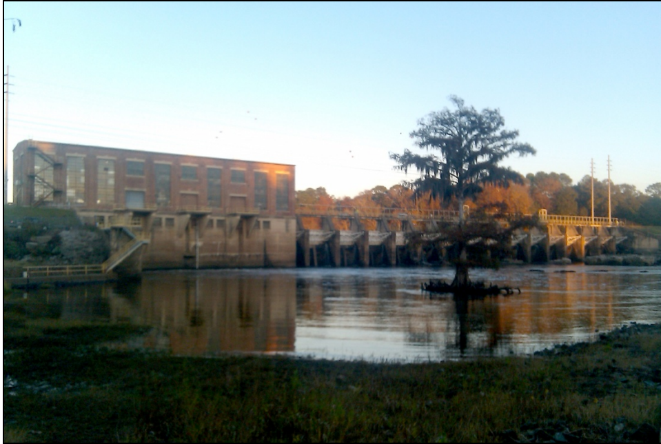
Figure 4-19. Flint River Dam
