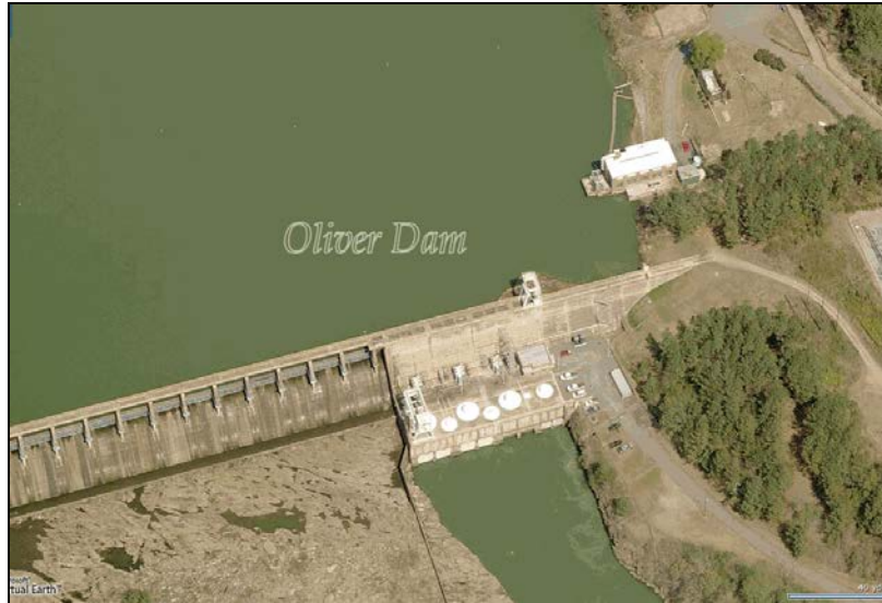
Figure 4-14. Oliver Dam (Photograph courtesy of GPC)
