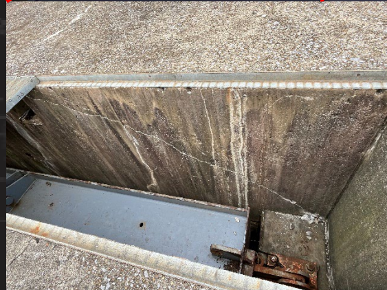
New Crack in Upstream Bulkhead Slot
