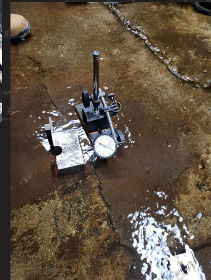
Crack in Machinery Room Floor
