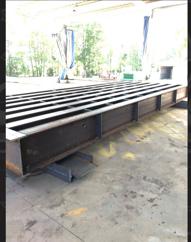
Bulkhead Section 1 Fit Up
