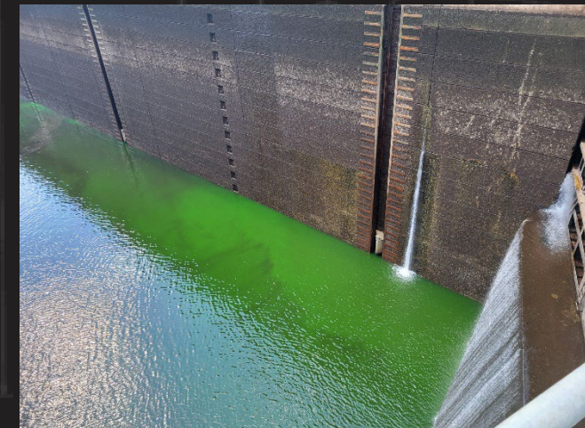
Dye Observed from Leaks in Lift Lines Along 14R
