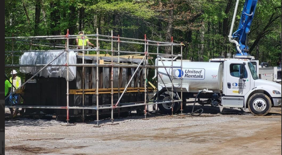
Wet concrete mix testing
