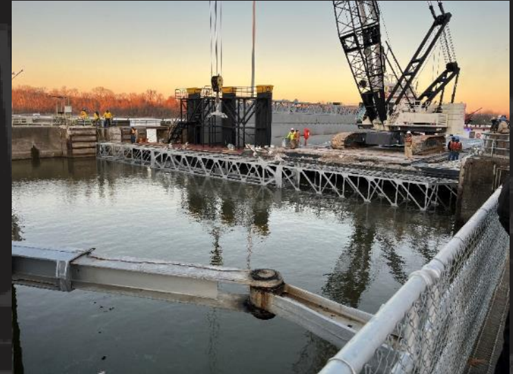
TVA Setting Upper Stoplogs
