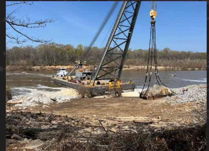
McKinney Salvage Debris Removal
