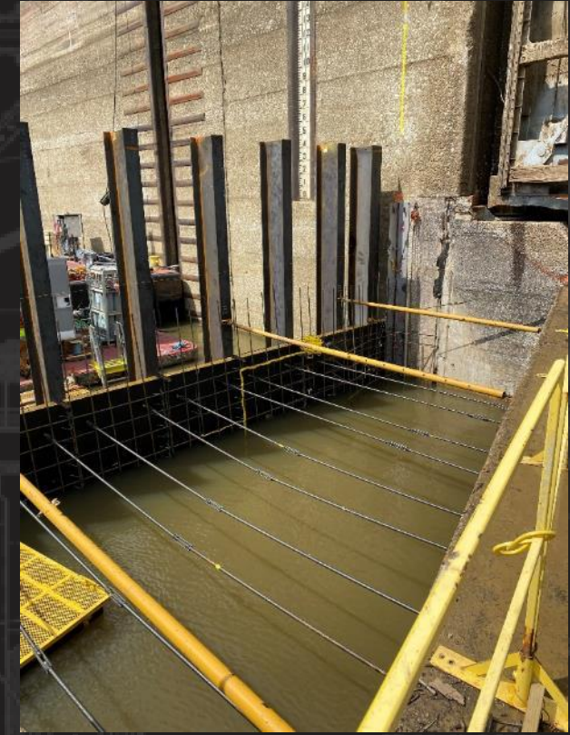
Installed Riverside Formwork
