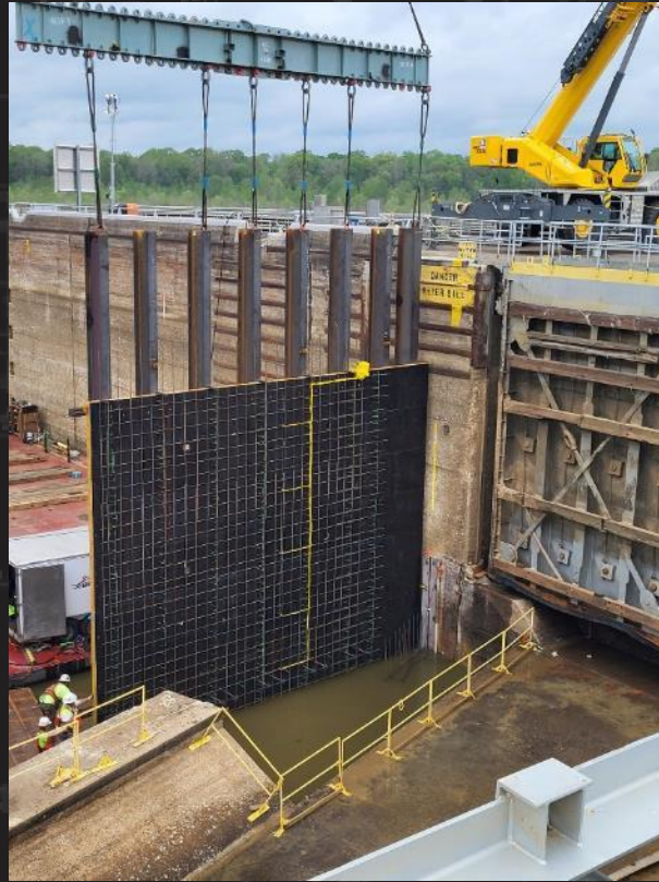
Installing Riverside Formwork
