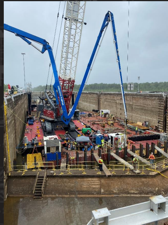
Concrete Placement on second monolith
