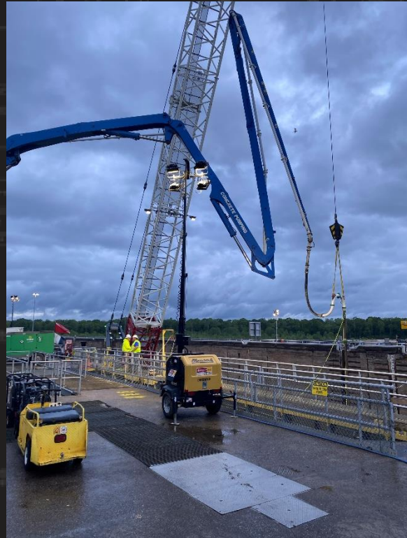
Concrete Placement on first monolith
