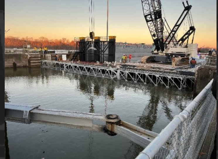
TVA Setting Upper Stoplogs
