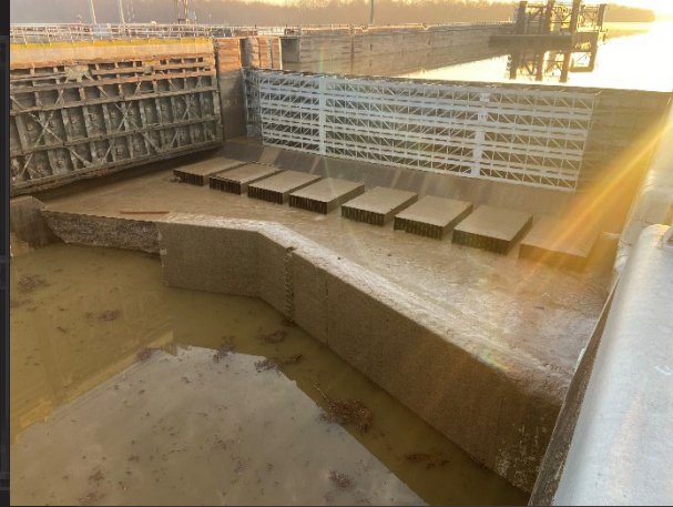
Damaged Sill
