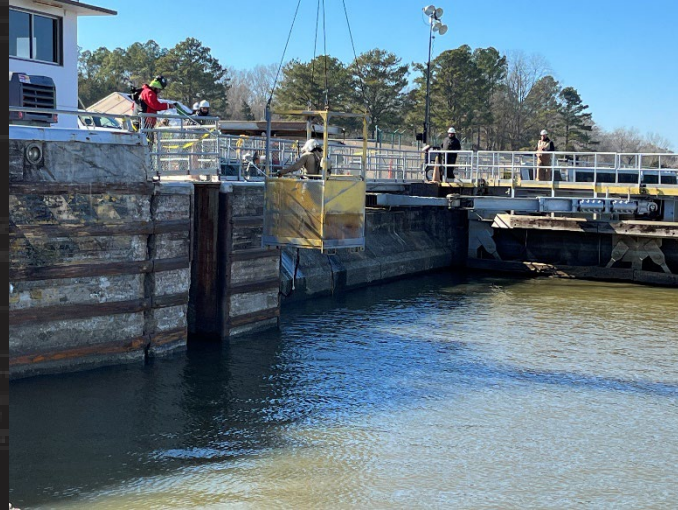
Diver Inspecting Stoplog Slot
