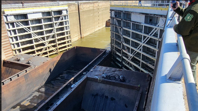
Lower Miter Gates Closing
