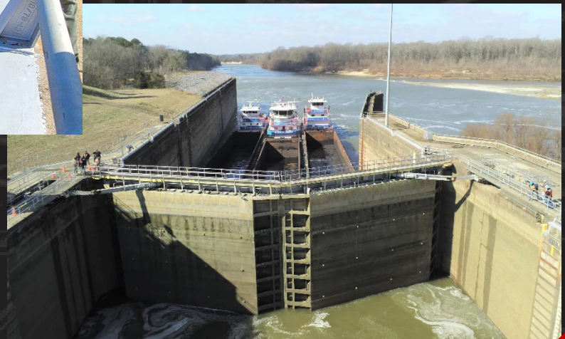
Lower Miter Gates Closed
