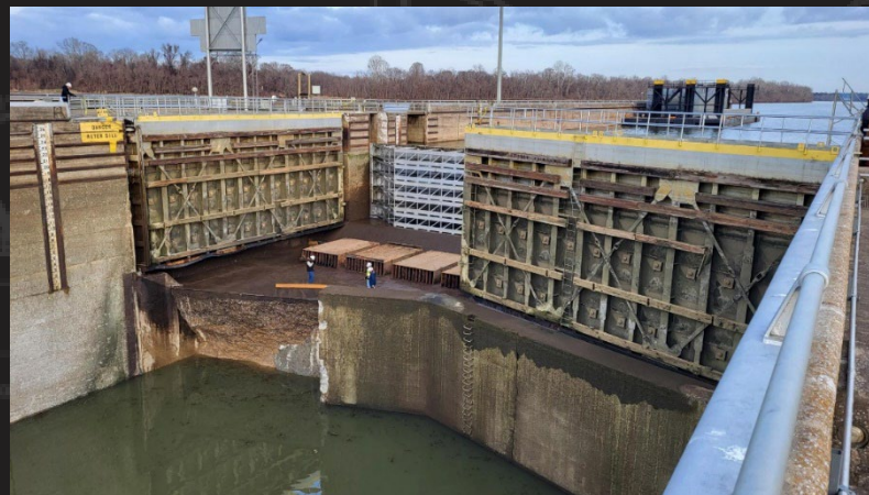
Upper Miter Gate Successful Operation
