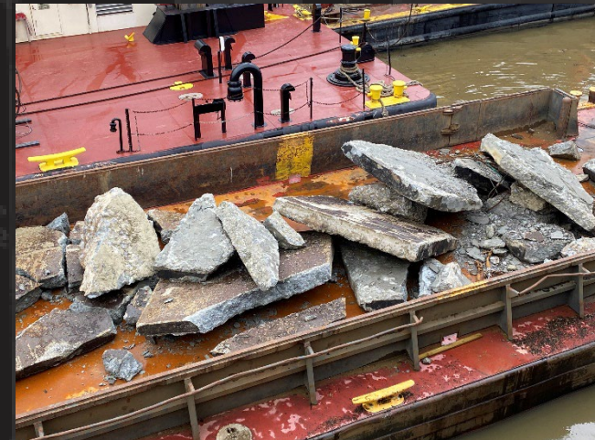
Concrete Debris Removal
