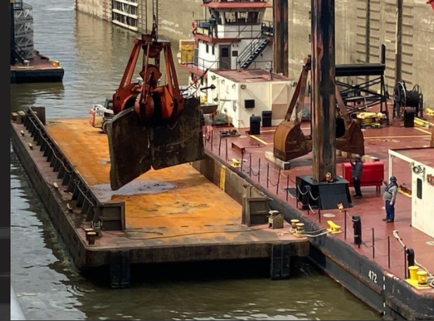
Floor Slab Debris Removal
