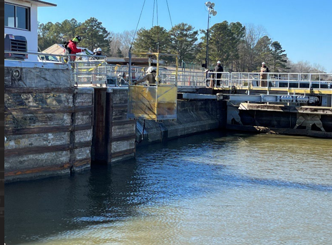
Diver Inspecting Stoplog Slot
