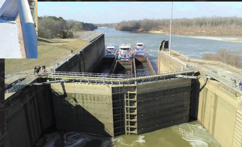
Lower Miter Gates Closed
