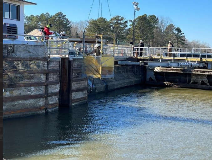
Diver Inspecting Stoplog Slot
