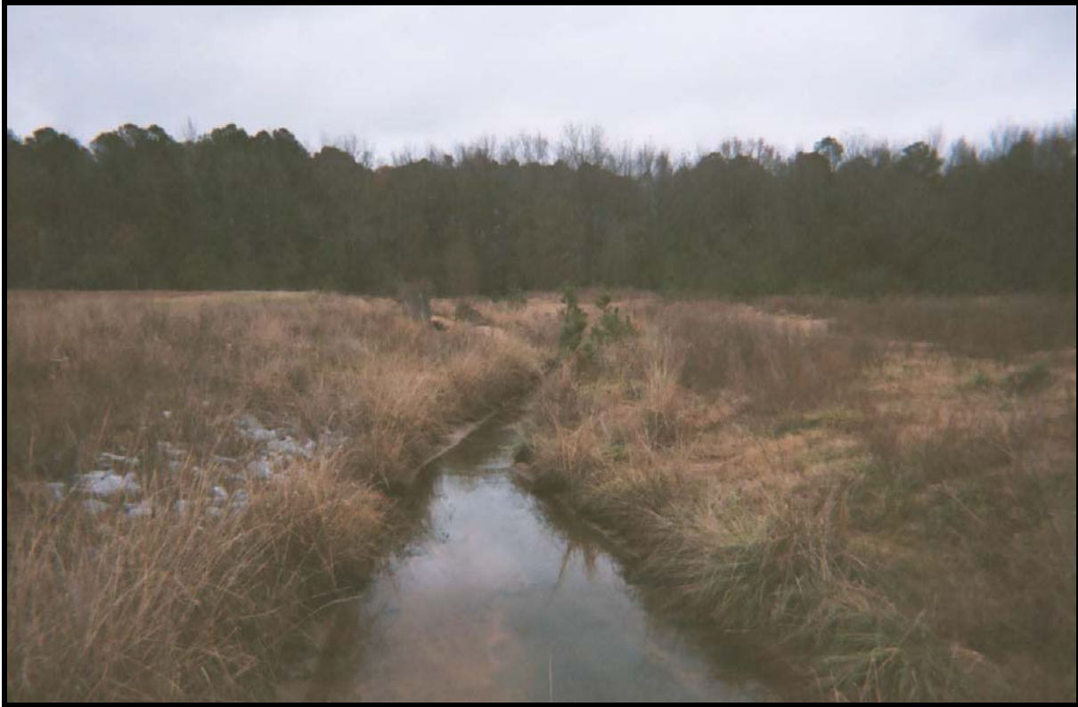
Photograph 3: Landfill No. 4 – Cement-lined ditch on fill area (facing east).
