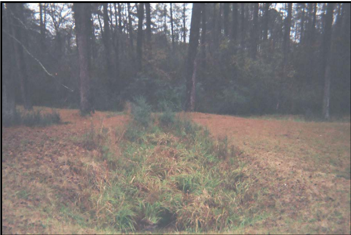
Photograph 20: Landfill No. 1 – A small drainage ditch located east of Coxwell Avenue. Empties into stream located behind trees.
