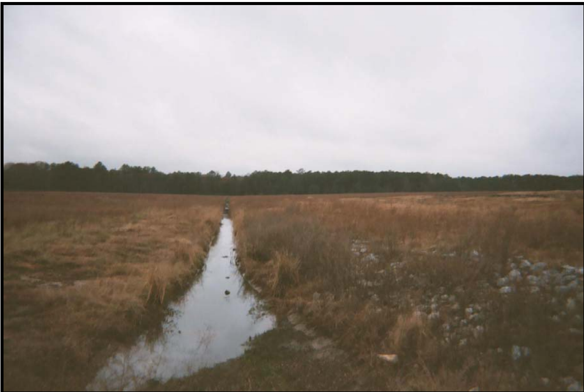
Photograph 2: Landfill No. 4 – Cement-lined ditch located on fill area (facing west).
