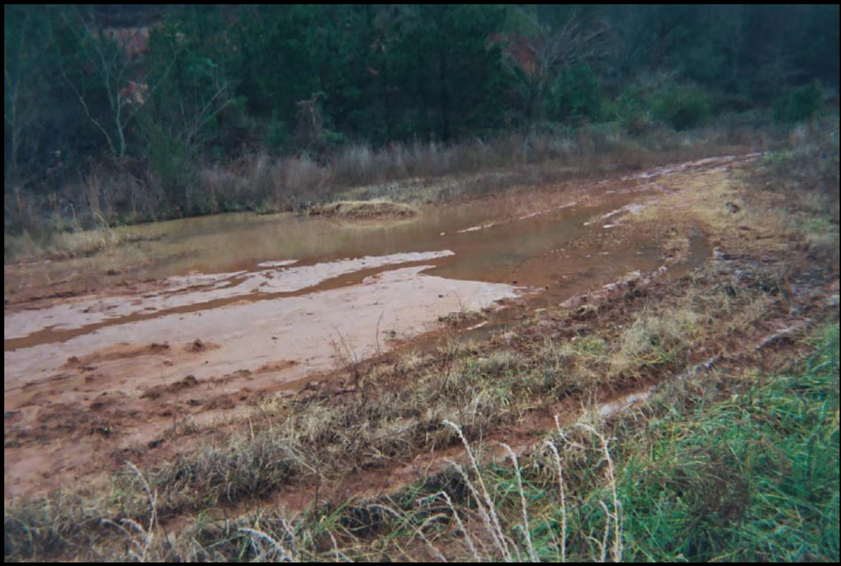
Photograph 9: Fill Area at Range 30 – Depressional area in road where water collects; some wetland vegetation present.
