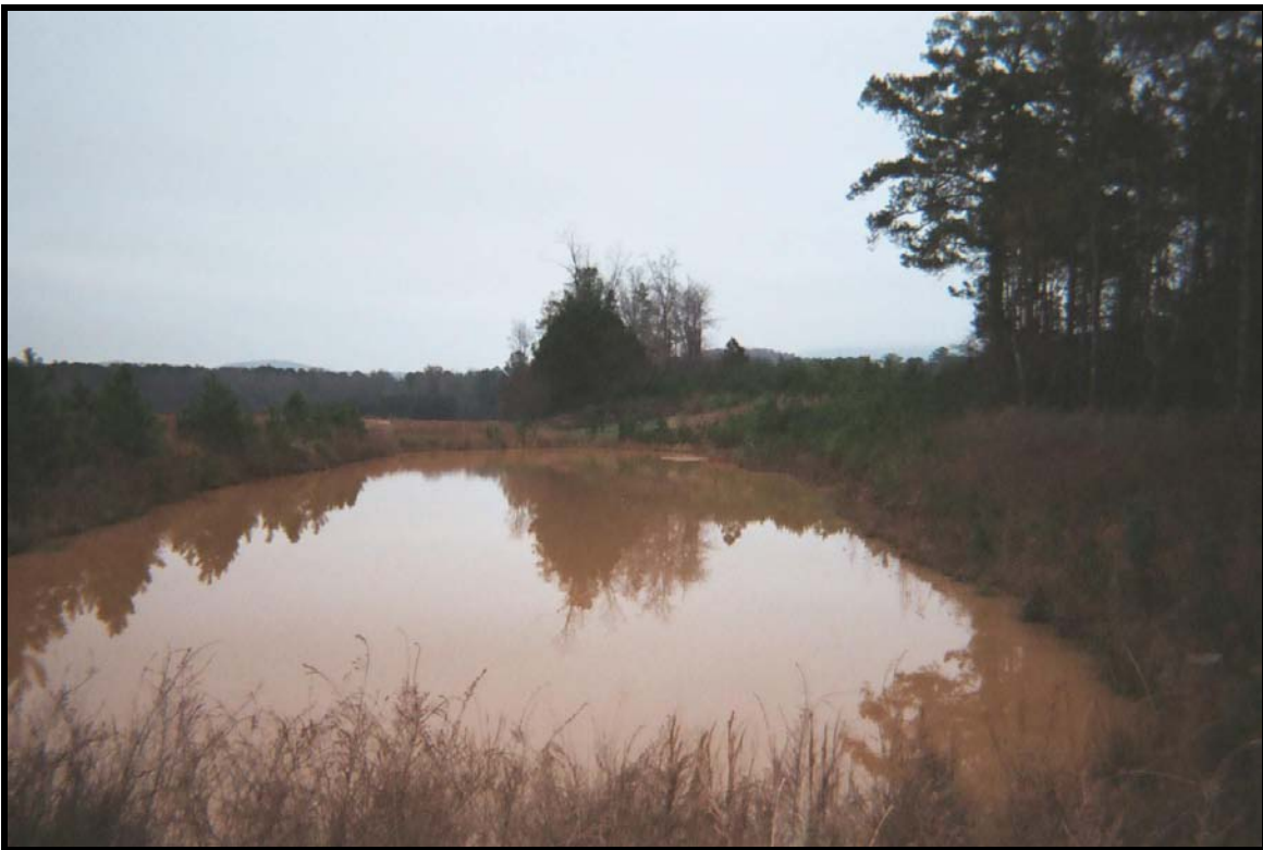
Photograph 6: Landfill No. 4 – Detention pond located in the southwest corner of landfill.
