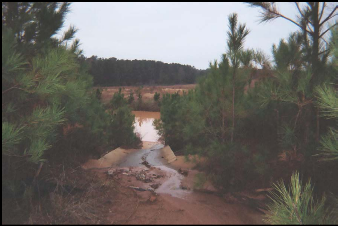
Photograph 7: Landfill No. 4 – Cement drainage-way leading into detention pond located at southwest corner of landfill.
