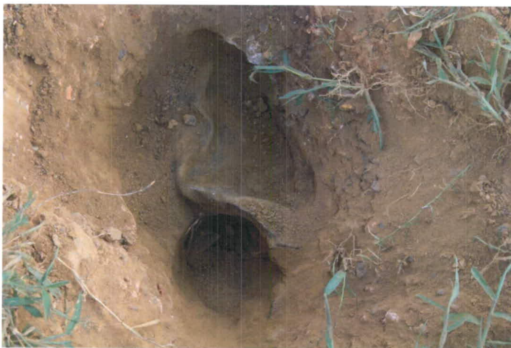
1) Crushed metal drums in hand excavation at planned location of VP-7 in TA-3.
