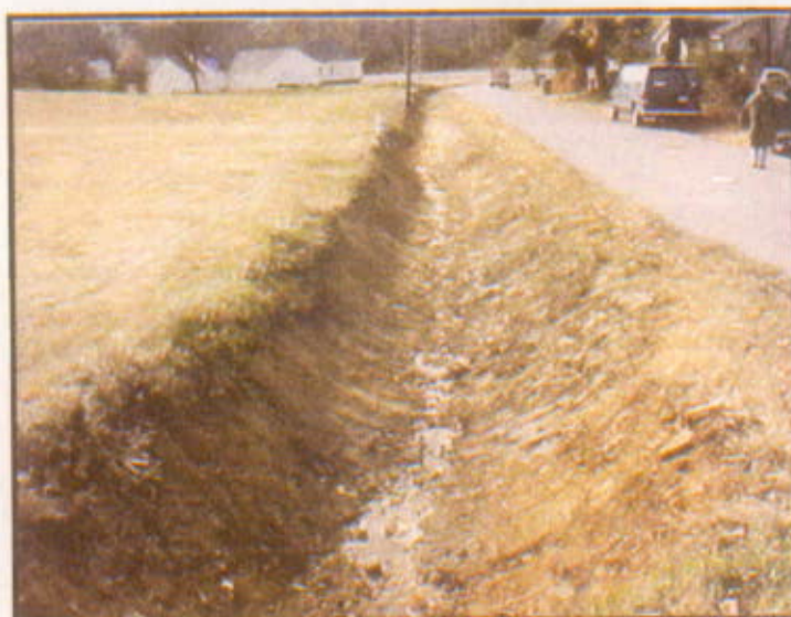
Photograph 1 Downstream view of Mullen Road Ditch
