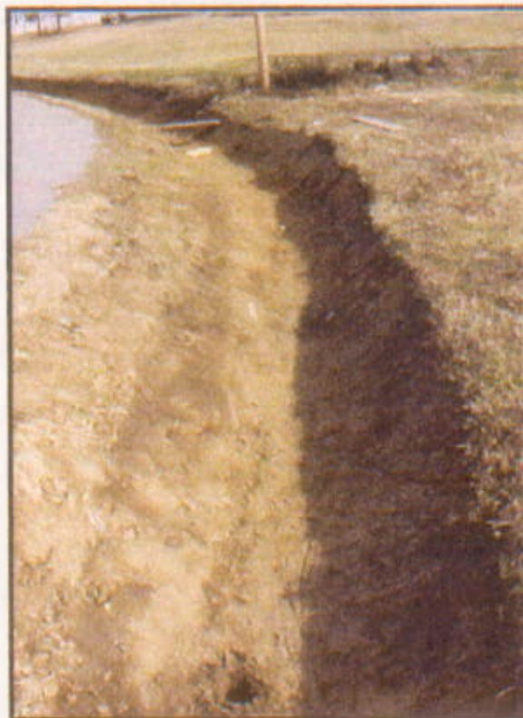
Photograph 4 Mullen ditch looking upstream to facility
