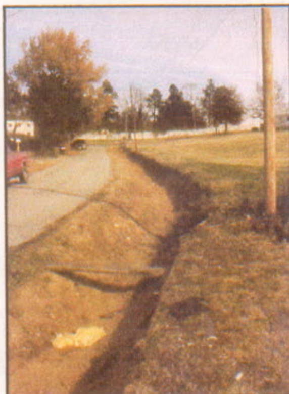
Photograph 5 Mullen Road Ditch
