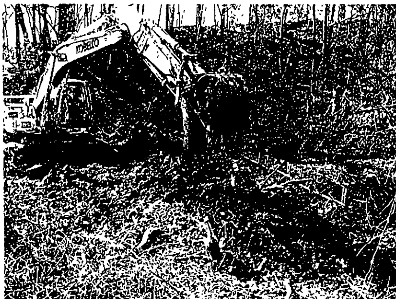
Clearing and Grubbing Vegetation
