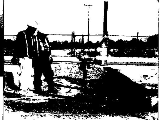
Workers complete the removal of the old railroad tracks from Dunn Road
