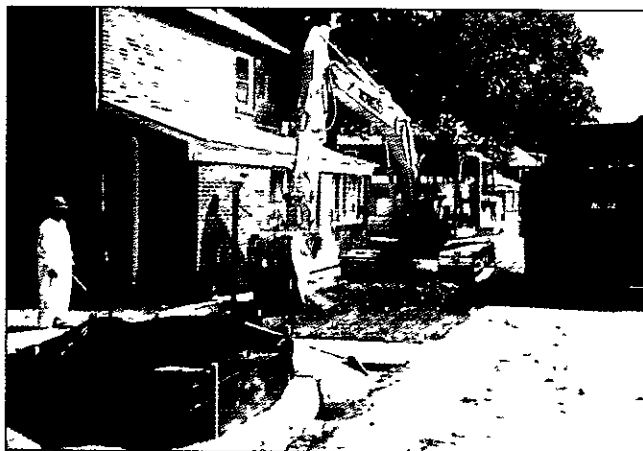
Environmental field staff with OHM Remediation remove surface soil from around the housing area at the Depot as part of the on-going cleanup activities.
