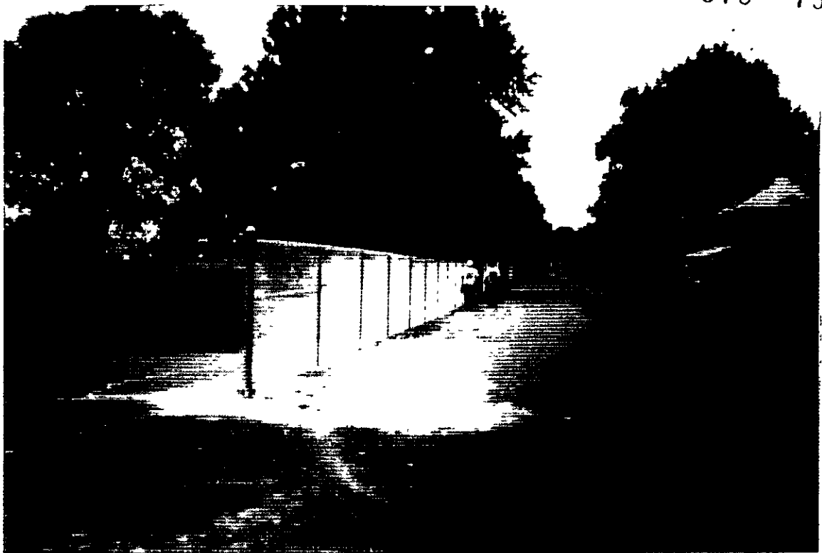
Date: 07/01/98 Description: INSTALLATION OF PERMANENT FENCE View Direction: NORTH
