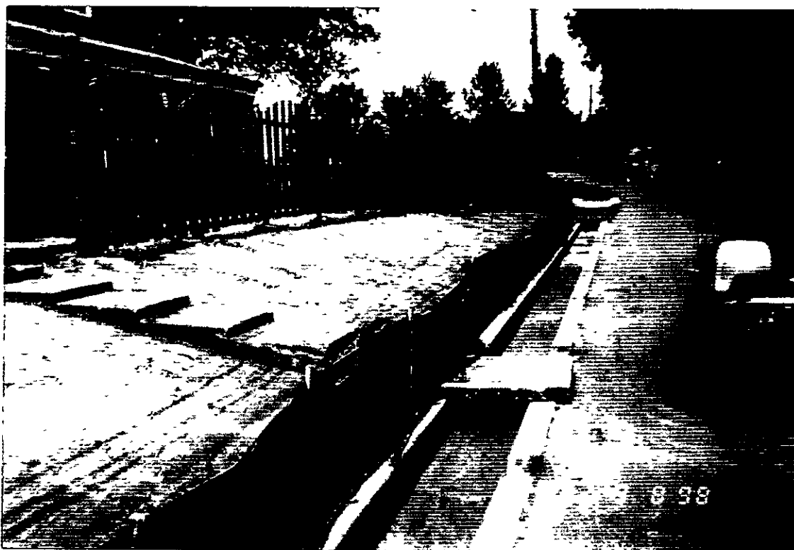
Date: 08/05/98 Description: AREA A AFTER EXCAVATION ACTIVITIES View Direction: NORTH
