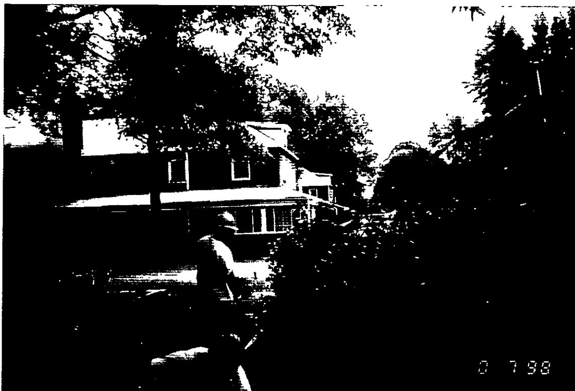
Date: 07/08/98 Description: CLEARING & GRUBING OF HOUSING AREA View Direction: SOUTH
