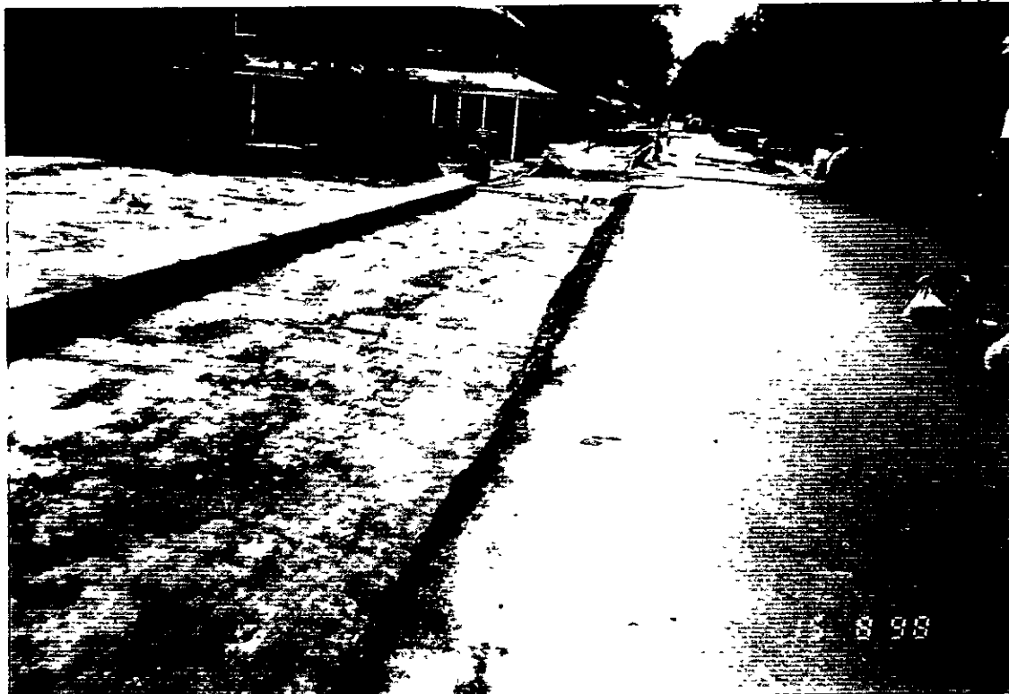
Date: 08/15/98 Description: EXCAVATING AREA B View Direction: SOUTH
