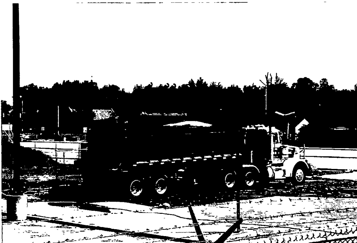
Date: 09/21/98 Description: LOAD OUT OF CONTAMINATED SOIL FOR OFF-SITE DISPOSAL View Direction: NORTHEAST
