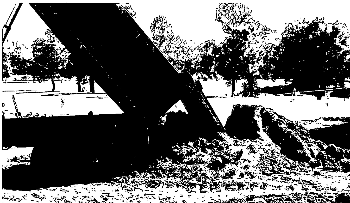
Date: 10/19/98 Description: BACKFILL MATERIALS BEING STAGED View Direction: SOUTHEAST
