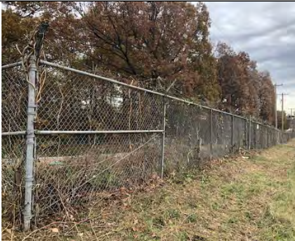
Western fence looking south. Barbed wire damaged in several places (Figure 1).
