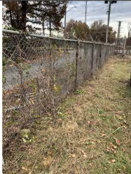
Western fence looking north where fence turns east. Fence post missing at left side of photo ( Location E , Figure 1). Barbed wire damaged in several places (Figure 1).
