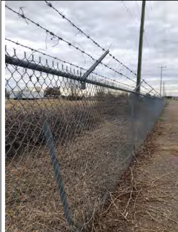
Eastern fence with broken fence post ( Location G , Figure 1).
