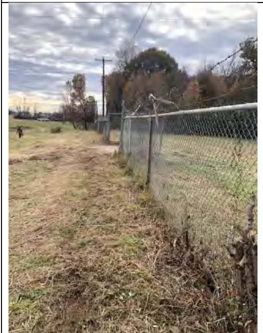
Western fence just north of gate looking south. Fence post missing ( Location C , Figure 1) and barbed wire in several places along top of fence is damaged (Figure 1).
