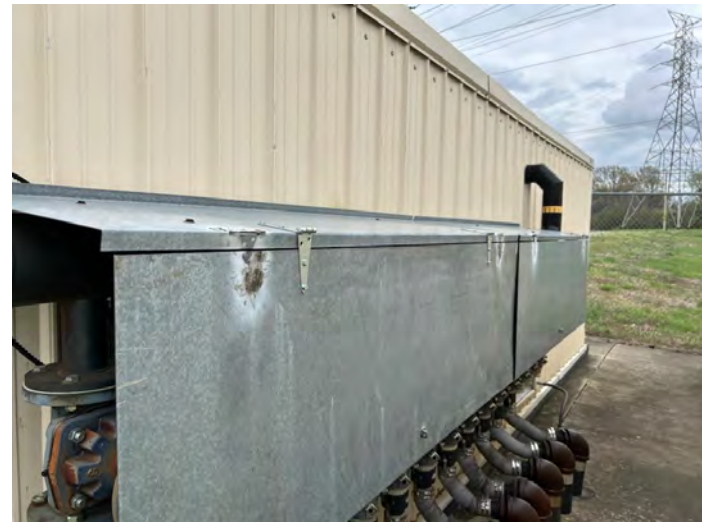
Valve Bank Cover after Repair
