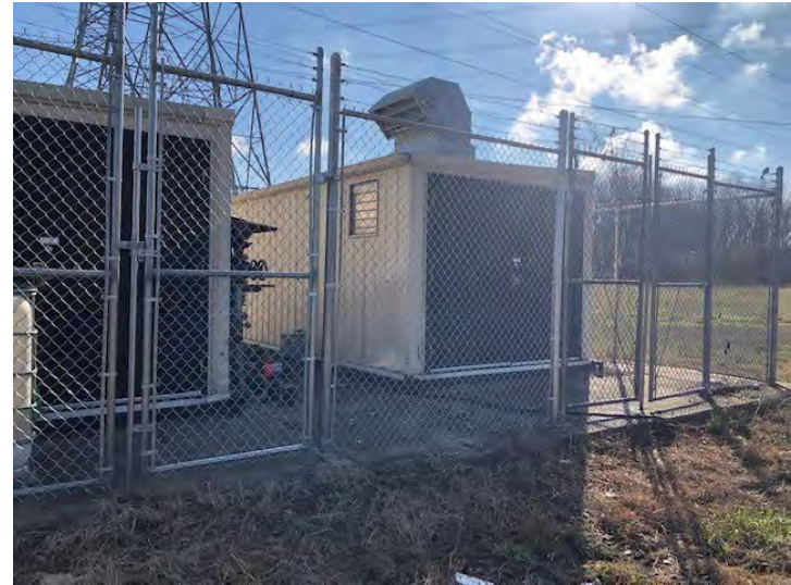
Fence and Gate Repaired
