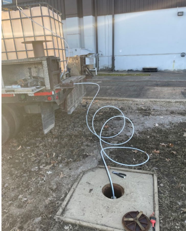
Photograph B-7. Redevelopment of MW-311 at Building 560 (General Purpose Warehouse) AOP1
