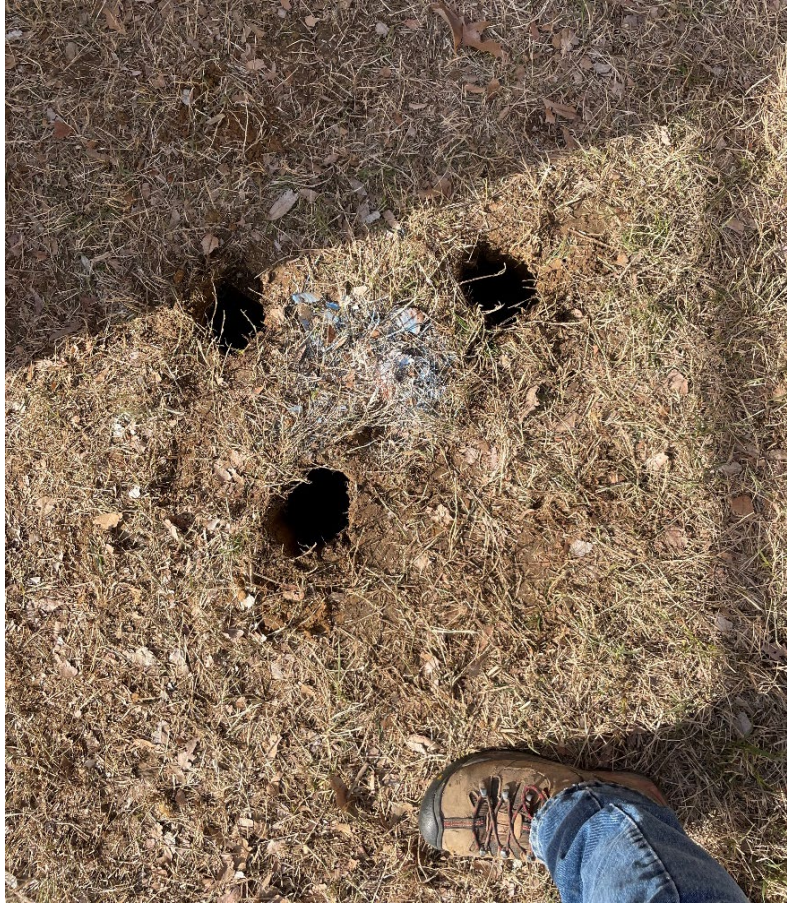
Photograph B-3. Example of Completed Borehole Clearance via Hand Augering at DDMT-529-01
