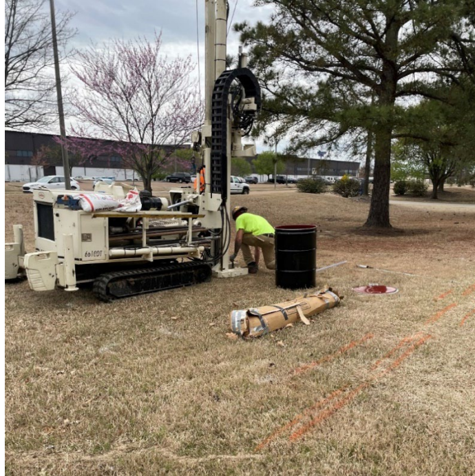
Photograph B-5. DPT Drilling at DDMT-550-01
