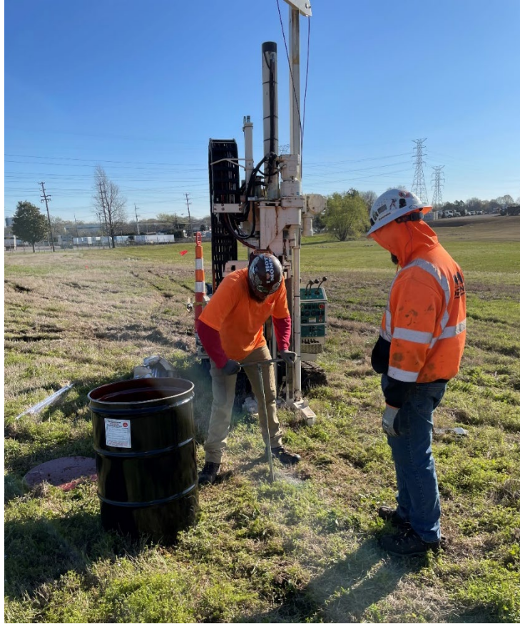
Photograph B-11. Hand Augering at DDMT-308-02
