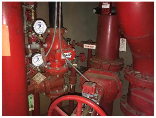
Photograph D-6. Water-based Fire Suppression
