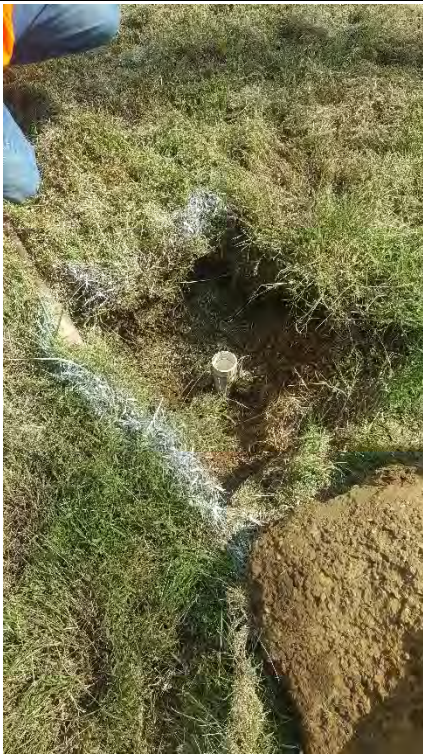
Photograph 9 ODAS-32 wellhead repair
