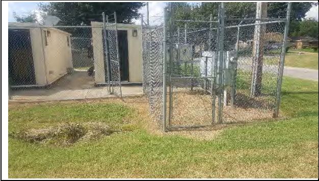
Photograph 19 Electrical compound vegetation cleared
