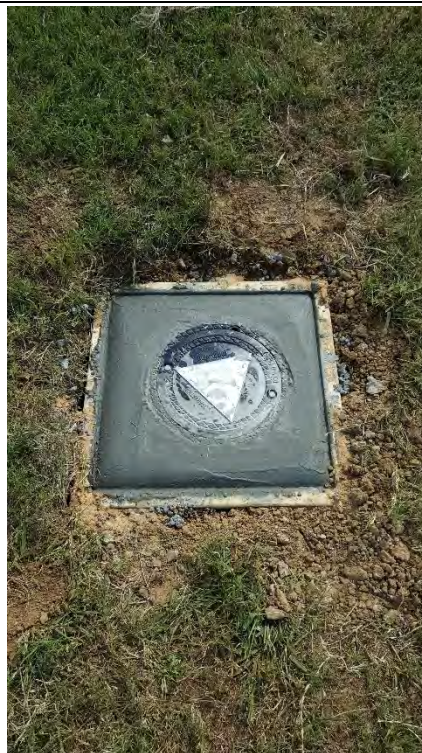
Photograph 12 ODAS-62 pad/vault replacement
