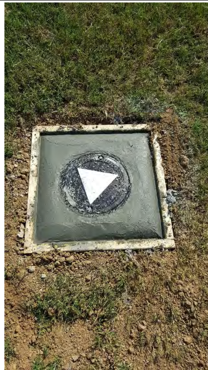
Photograph 8 ODAS-74 pad/vault replacement
