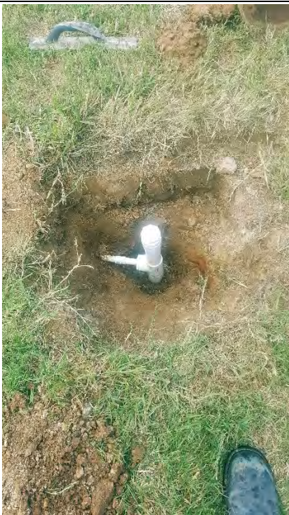
Photograph 11 ODAS-62 wellhead repair
