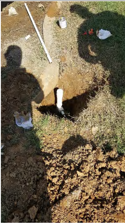
Photograph 5 ODAS-17 wellhead repair
