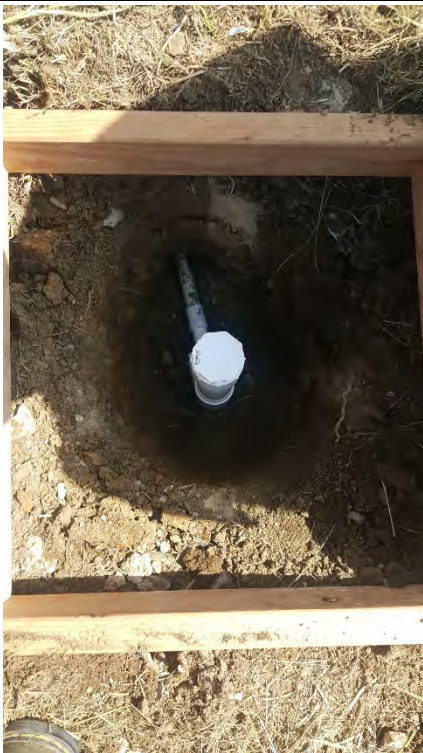
Photograph 7 ODAS-05 wellhead repair
