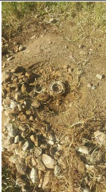
Photograph 2 ODSVE-02 wellhead condition
