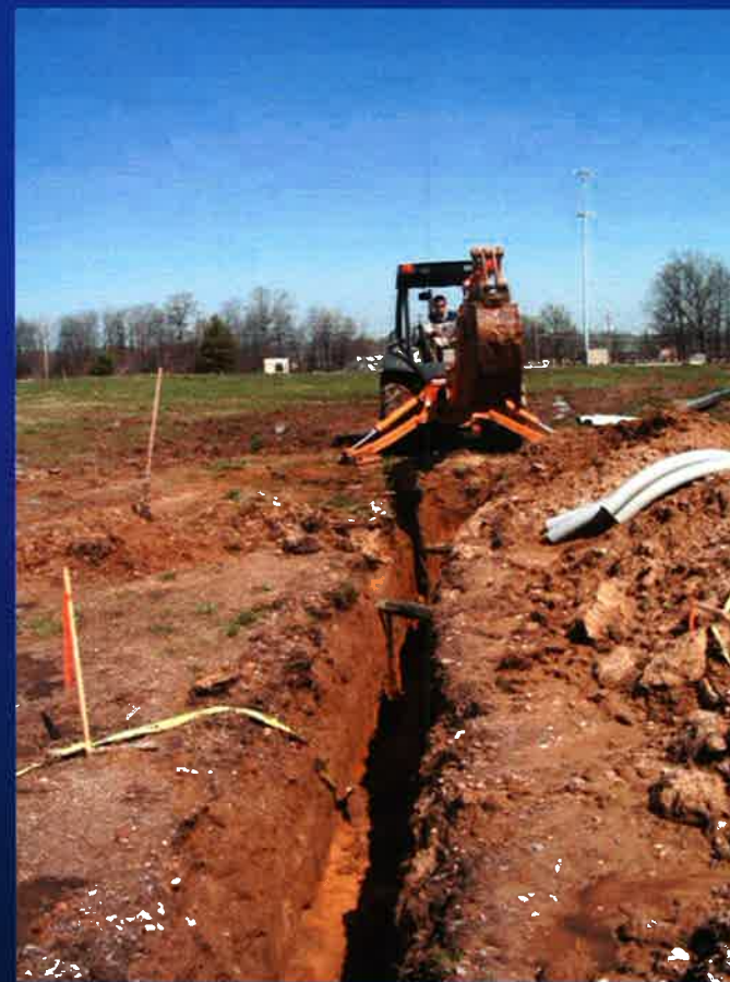
Installation of electrical conduit for thermal SVE.
