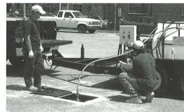
The Depot's environmental contractors operate the sodium lactate injection system that is being used to treat groundwater beneath the Main Installation.
