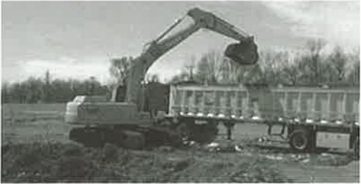
Environmental contractors loaded hazardous material from Disposal Site 3 into a lined container for shipment to an appropriate disposal facility.
