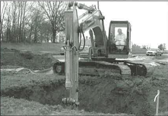
A Mactec field team member excavates affected soil from a former disposal site on Dunn Field.
