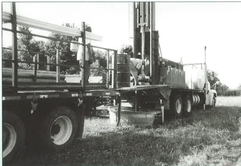
New groundwater monitoring wells have been installed in the Depot community to help gather data needed to design the cleanup remedy for groundwater at Dunn Field.
