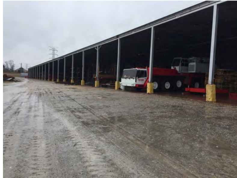
Building 1089 is concrete slab foundation on grade with no sumps or basements, open on one side
