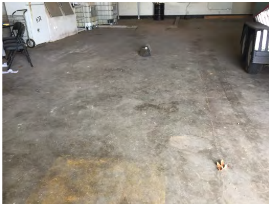
Building 265 shop/warehouse areas have concrete floors.
