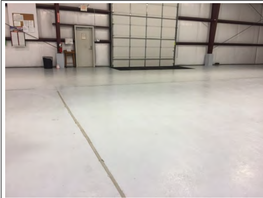
Building 970 Coated concrete floor in enclosed portion of Building 970.
