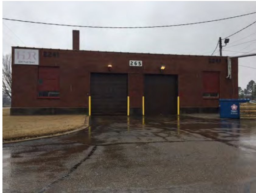
Building 265. Foundation is slab on grade and has no sumps or basement.
