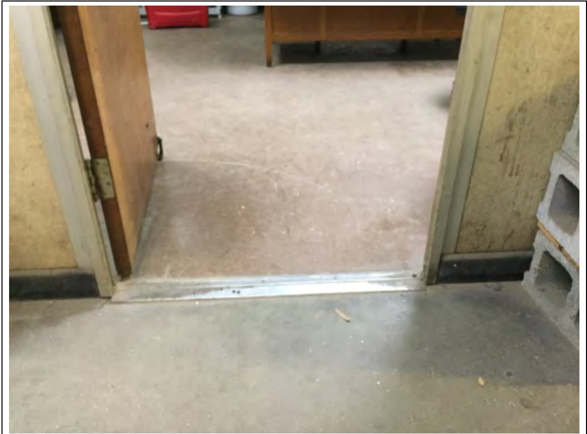
Building 265 has tiled office floors.
