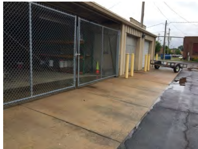
Storage overhang connected to south side of Building 260/261. This section shed was added after property transfer and is not part of the original structure.
