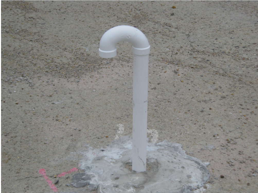
Photograph 5: P-traps were installed on new SVE wells to keep out rain and dirt/debris. P-traps can be removed to attach wells to conveyance piping via flexible hose.
