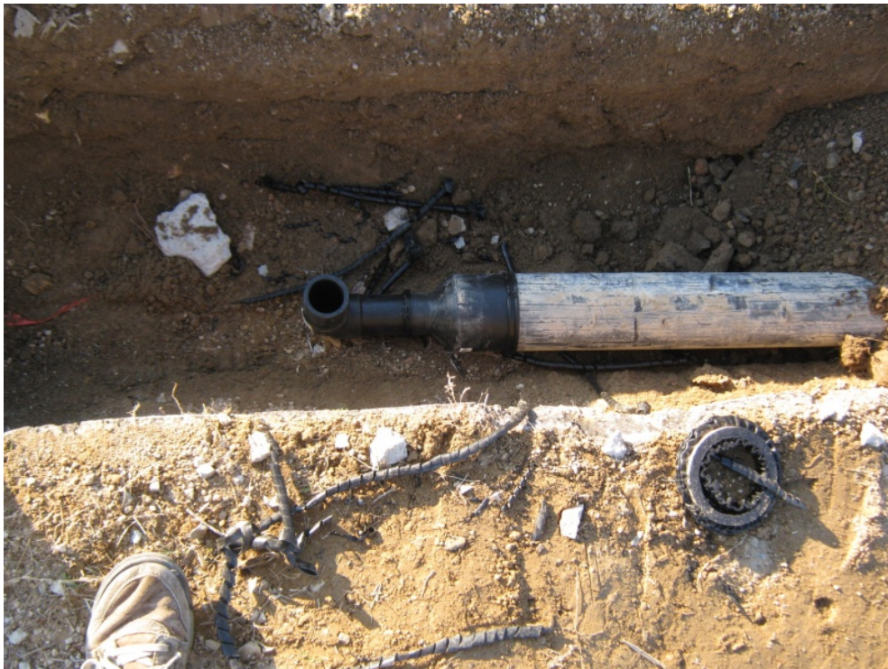
Photograph 2: Four-inch conveyance line with reducing fitting and elbow attached.
