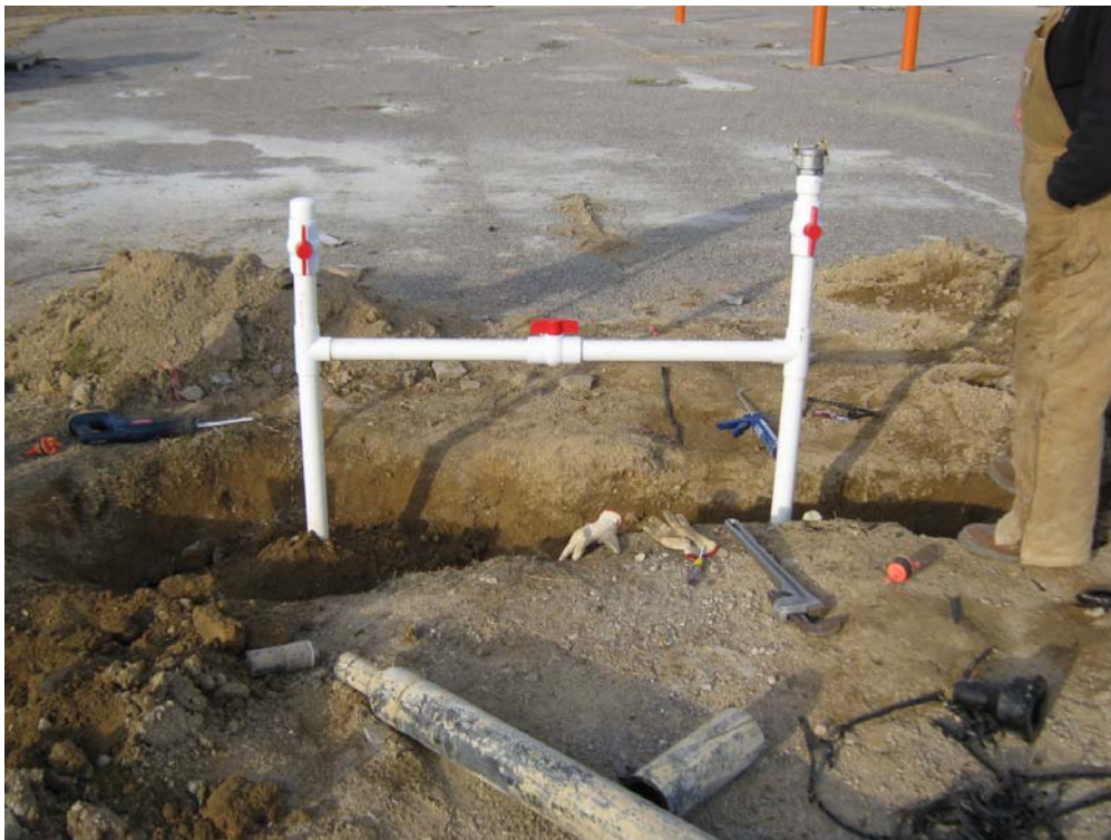
Photograph 4: Finished connection. SVE well is on the left. Valves on each line and fitting on conveyance line riser to connect new SVE wells.
