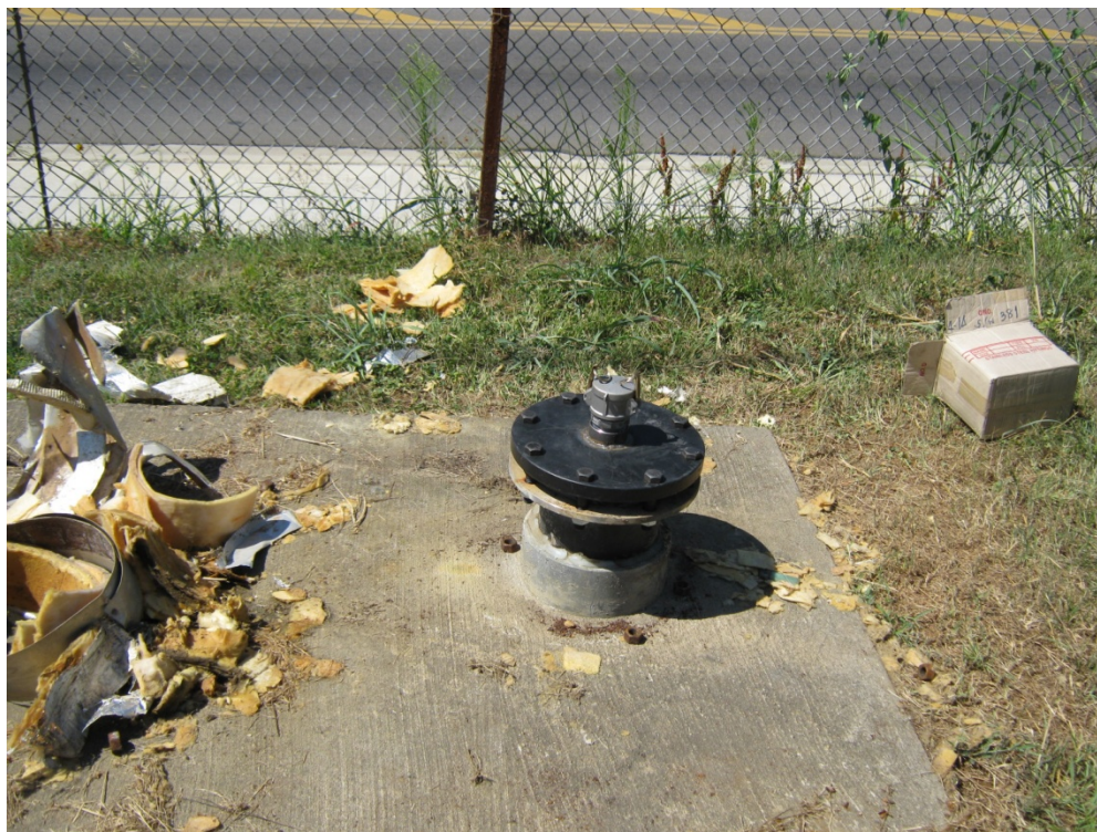
Photograph 11 - A cam-lock was added the sewer discharge to facilitate disposal of waste water generated during remedial action operations and monitoring.
