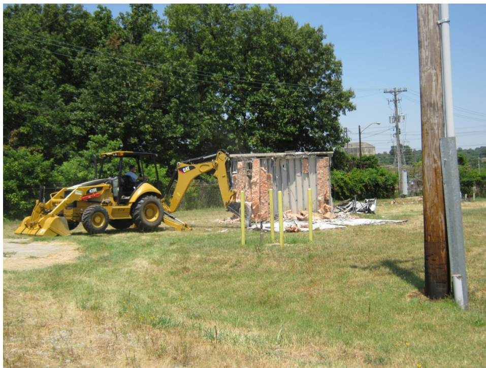
Photograph 9 - The control building was demolished; the electrical components were removed for recycling.
