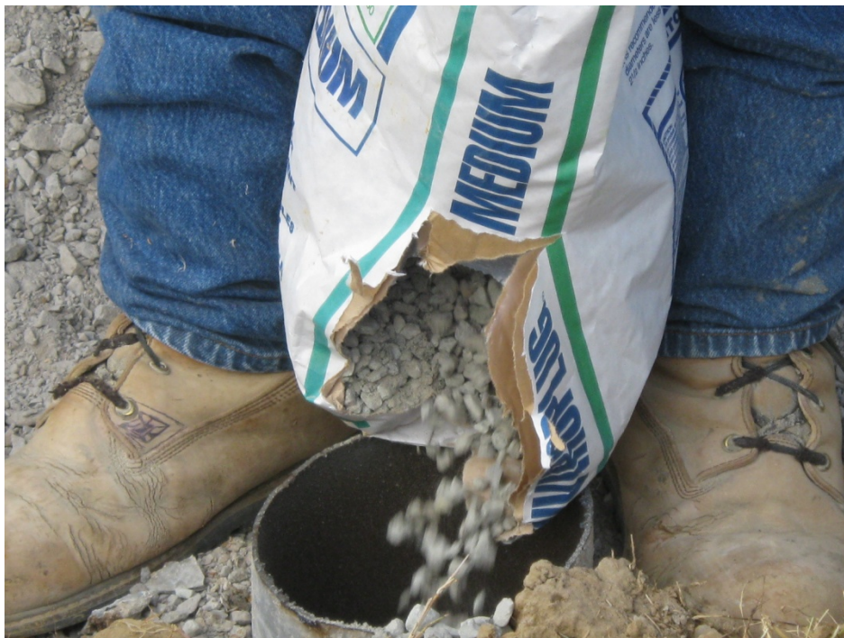
Photograph 13 - Bentonite chips were added to seal the screened section and minimize waste water generated during grouting.
