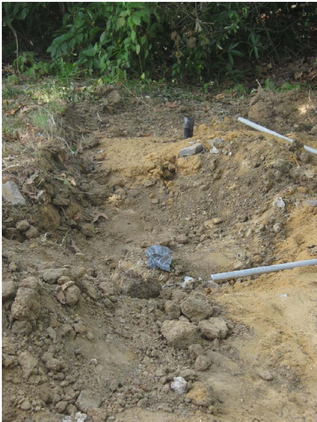
Photograph 12 - After well houses and pads were removed, the soil was excavated and the steel well casing was cut off about 1 foot below ground surface. The casing was covered with duct tape until abandonment. The excavated soil was replaced during site restoration.
