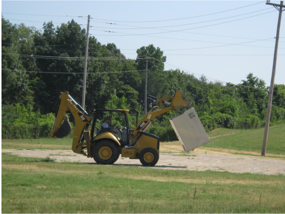
Photograph 7 - Contractors started by removing well housings and staged them on the asphalt pad at Dunn Field.
