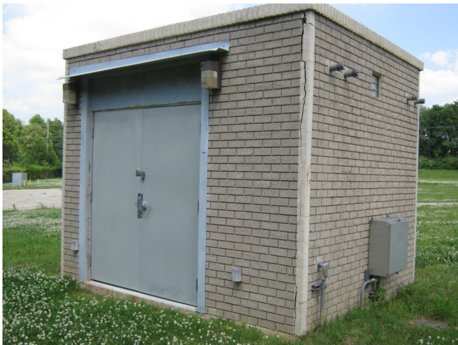
Photograph 1 – IRA Control Building
