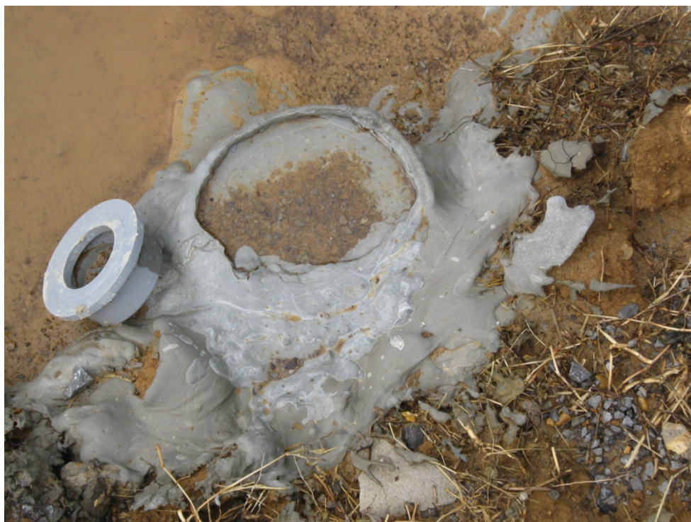
Photograph 14 - The wells were grouted to the top of casing.
