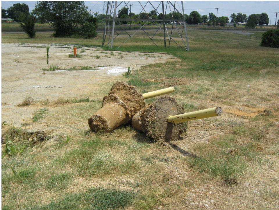
Photograph 8 - After IRA housings were removed, the bumper posts and the pads were removed.
